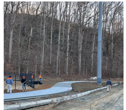
SPRINGWAY TRAIL - RIVER PARK
