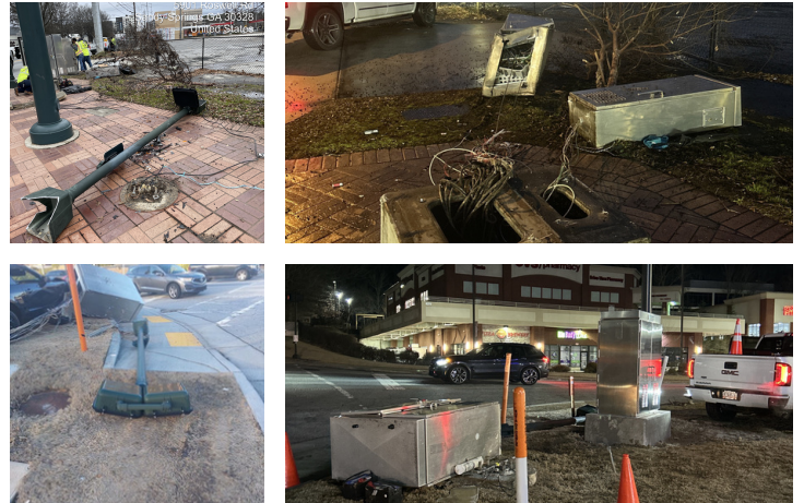
CABINET DAMAGE FROM MOTOR VEHICLE ACCIDENTS
