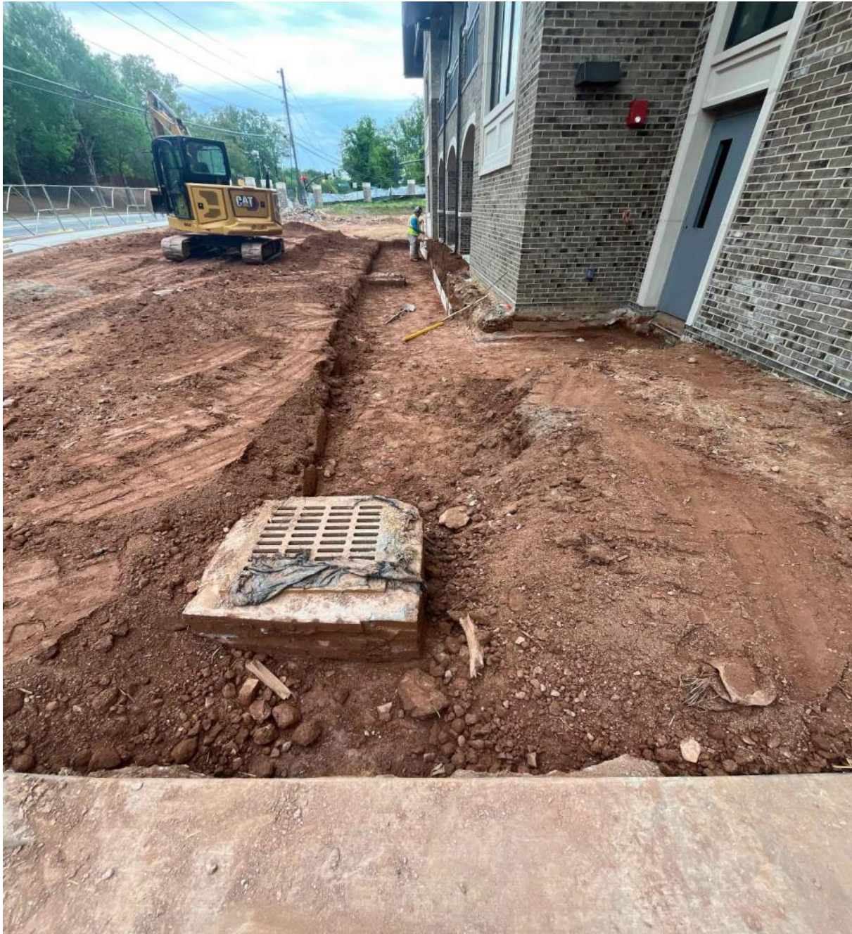
Preparing Subgrade at For Permeable Paver Installation at Spalding Elevation
