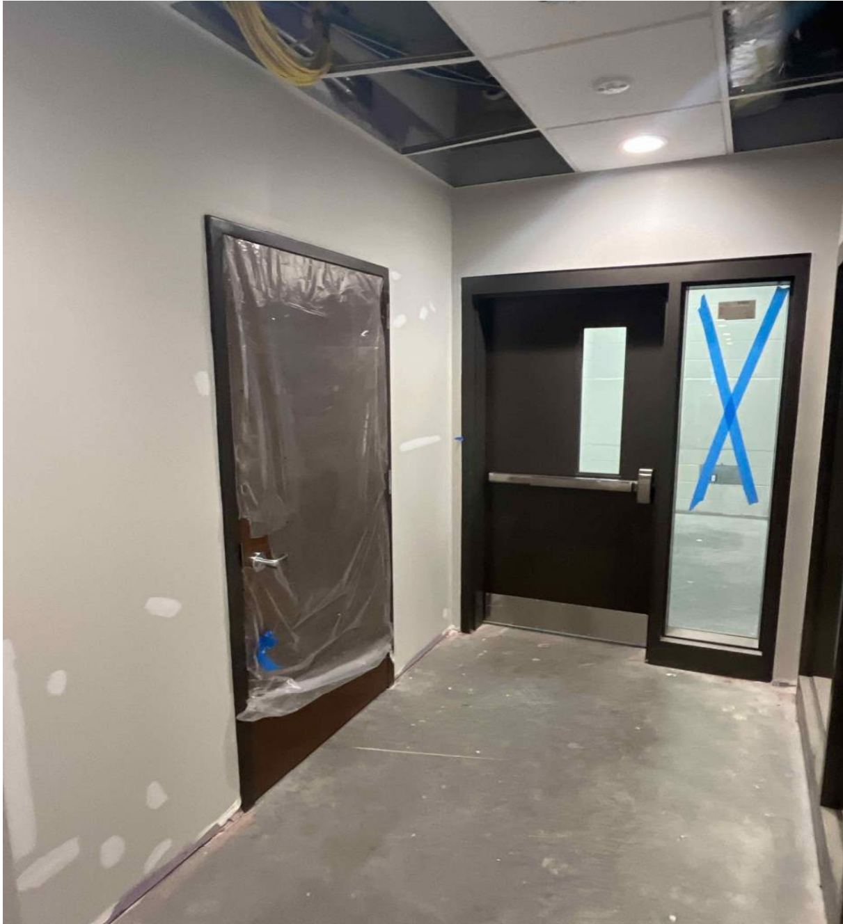
Installation of Interior Wood Doors and Hardware at the Second Floor
