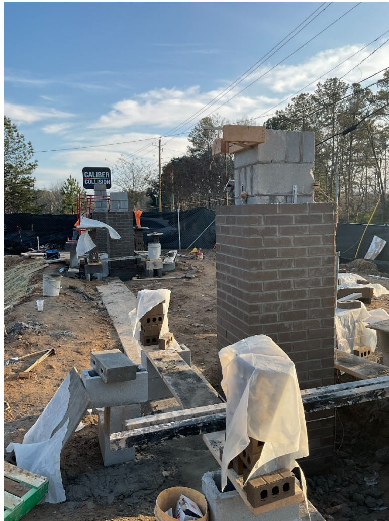
Began Brick Columns' Construction
