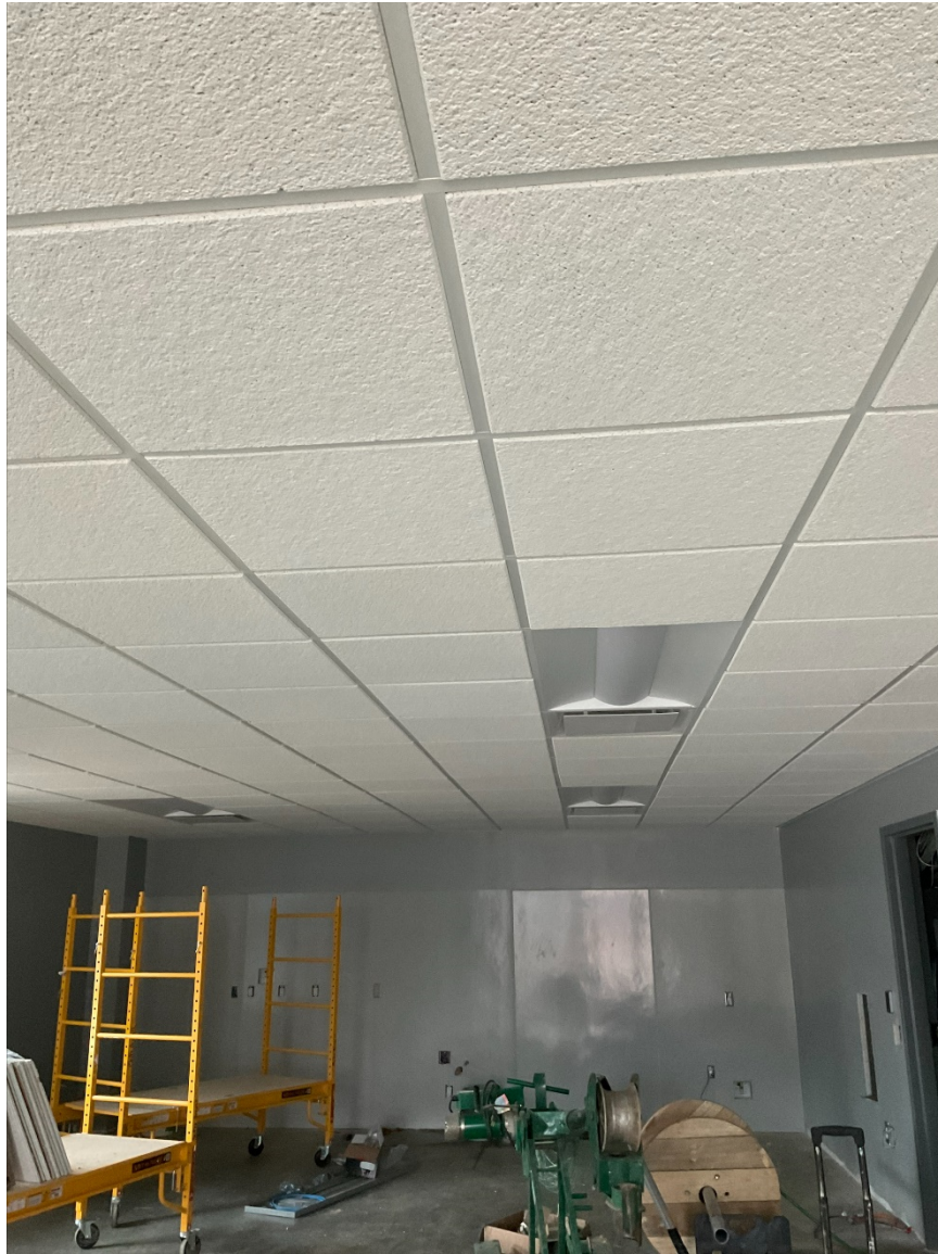
Ceiling Grid Installed In Office
