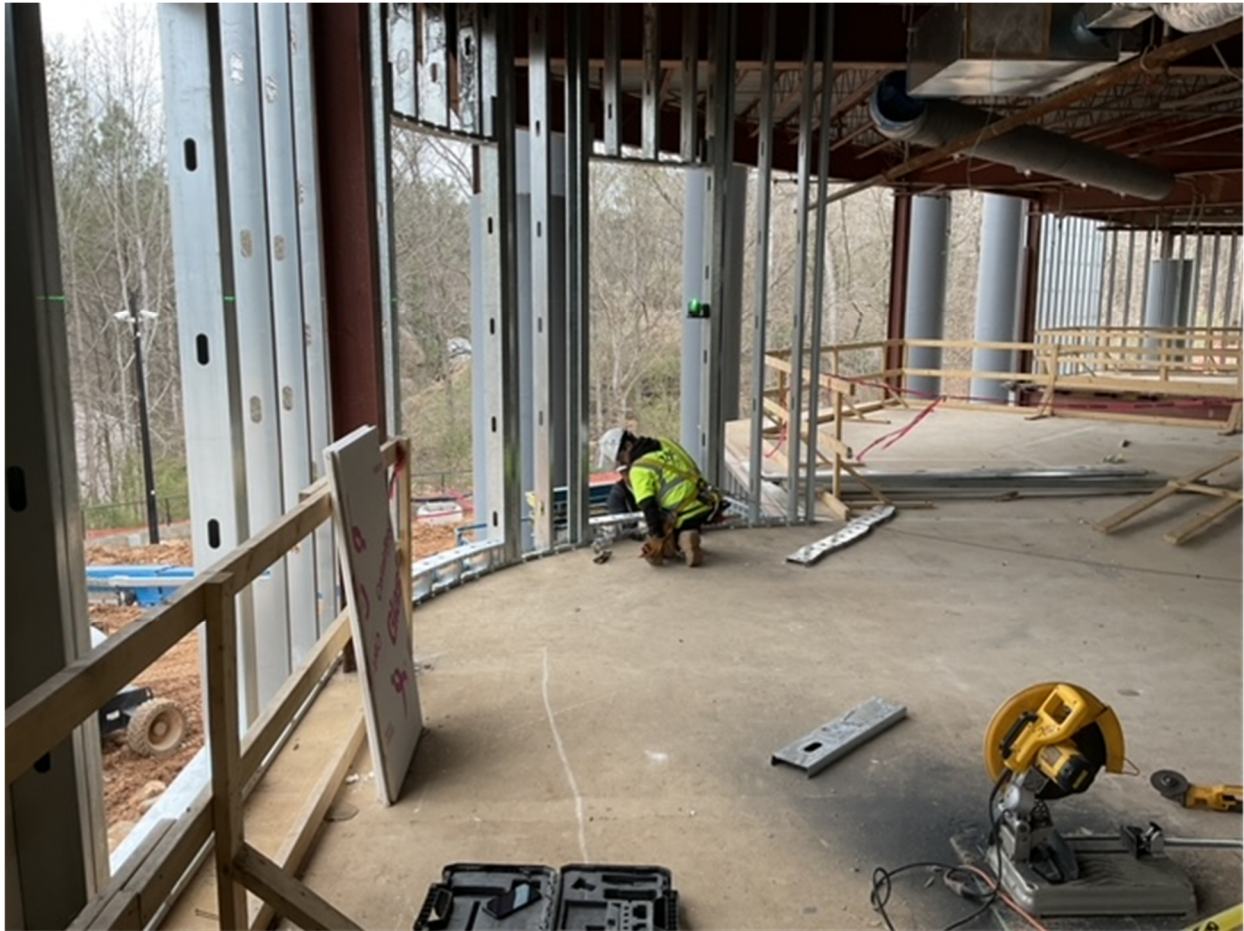
Setting Window Frames
