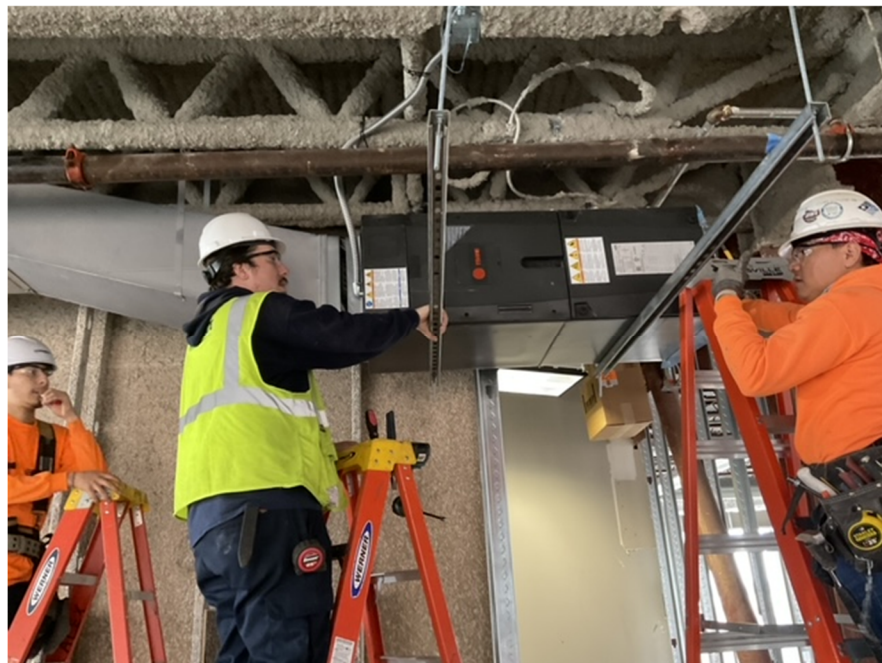
O/H & In Wall Plumbing Rough-In
