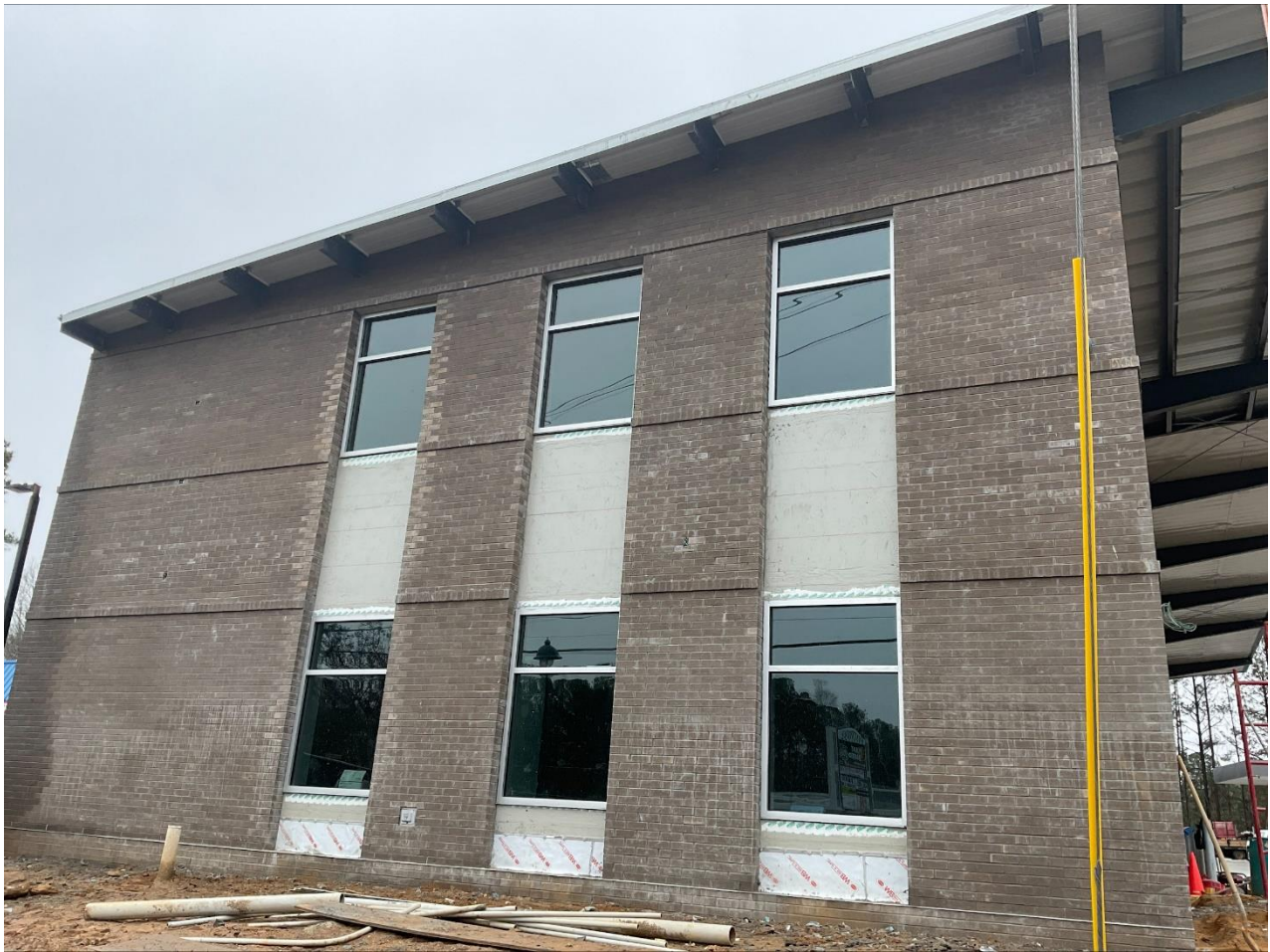
Brick On The Building Completed
