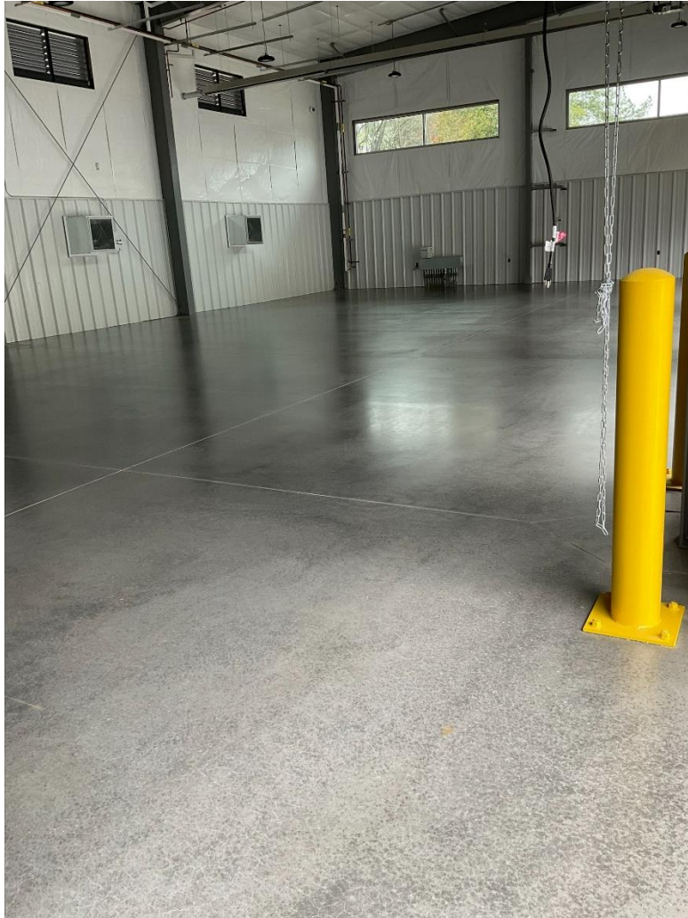
Floors Sealed In Office And Shop Area
