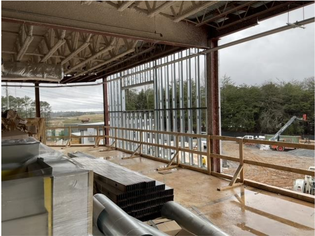
Setting Window Frames/Framing
