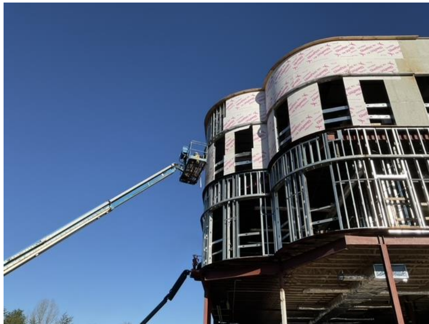
Exterior Framing/Sheathing
