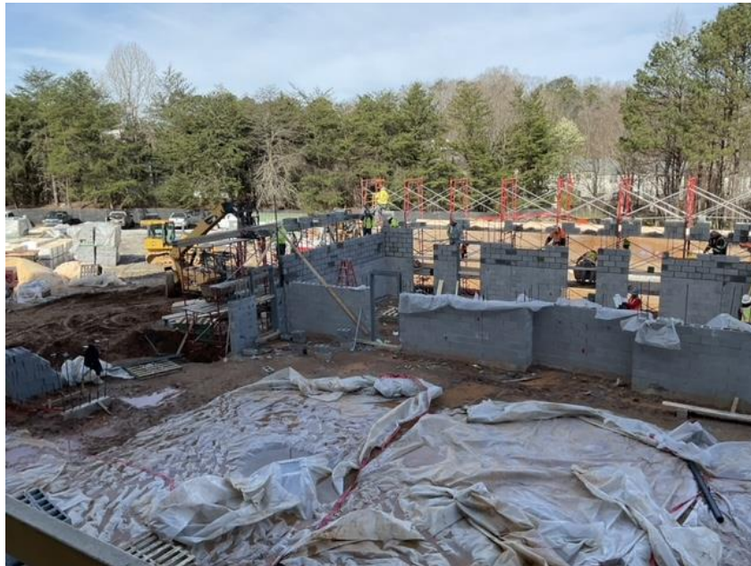
CMU Walls at Addition C
