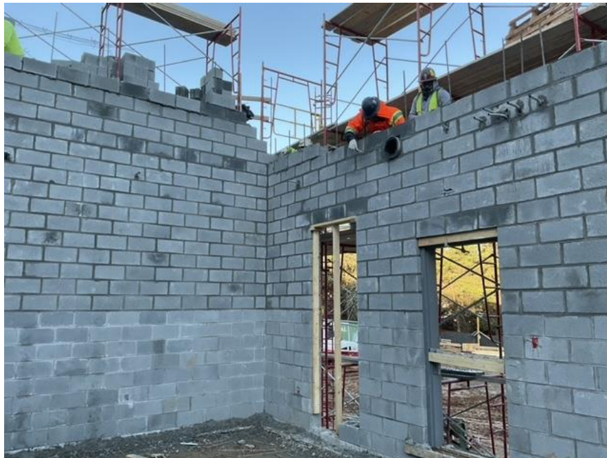
CMU Walls at Addition C
