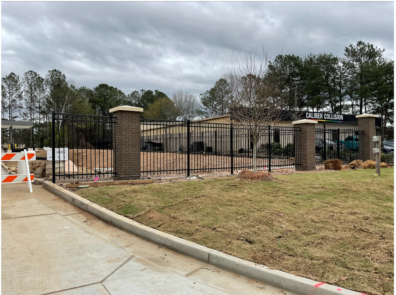
Fencing Installed Around Site
