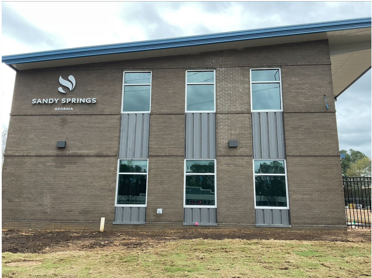
Building Signage Installed
