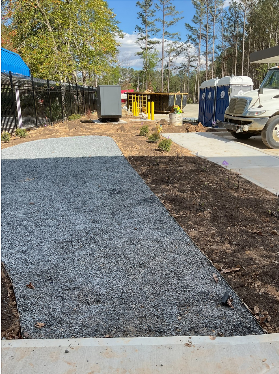
Continued Work On Hardscapes And Landscapes
