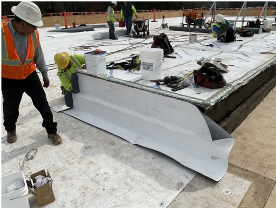
New Roof Install
