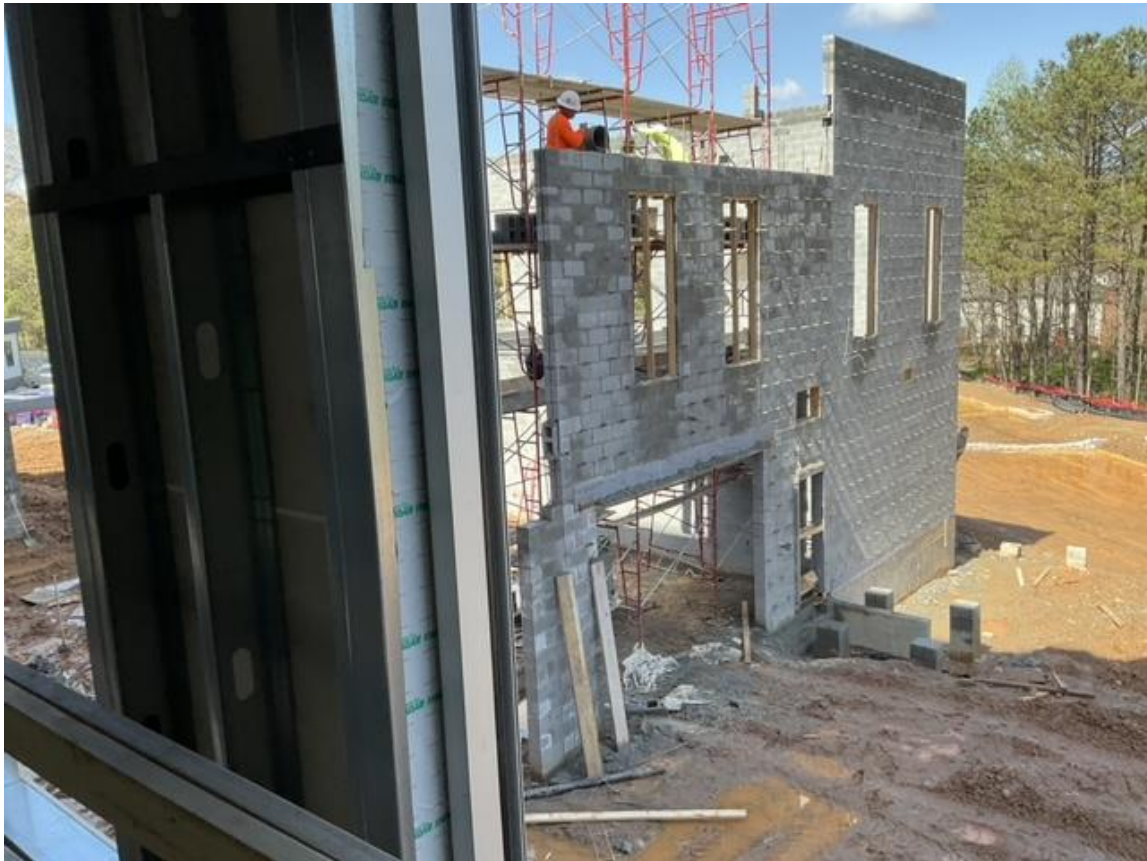
CMU Wall at Sallyport
