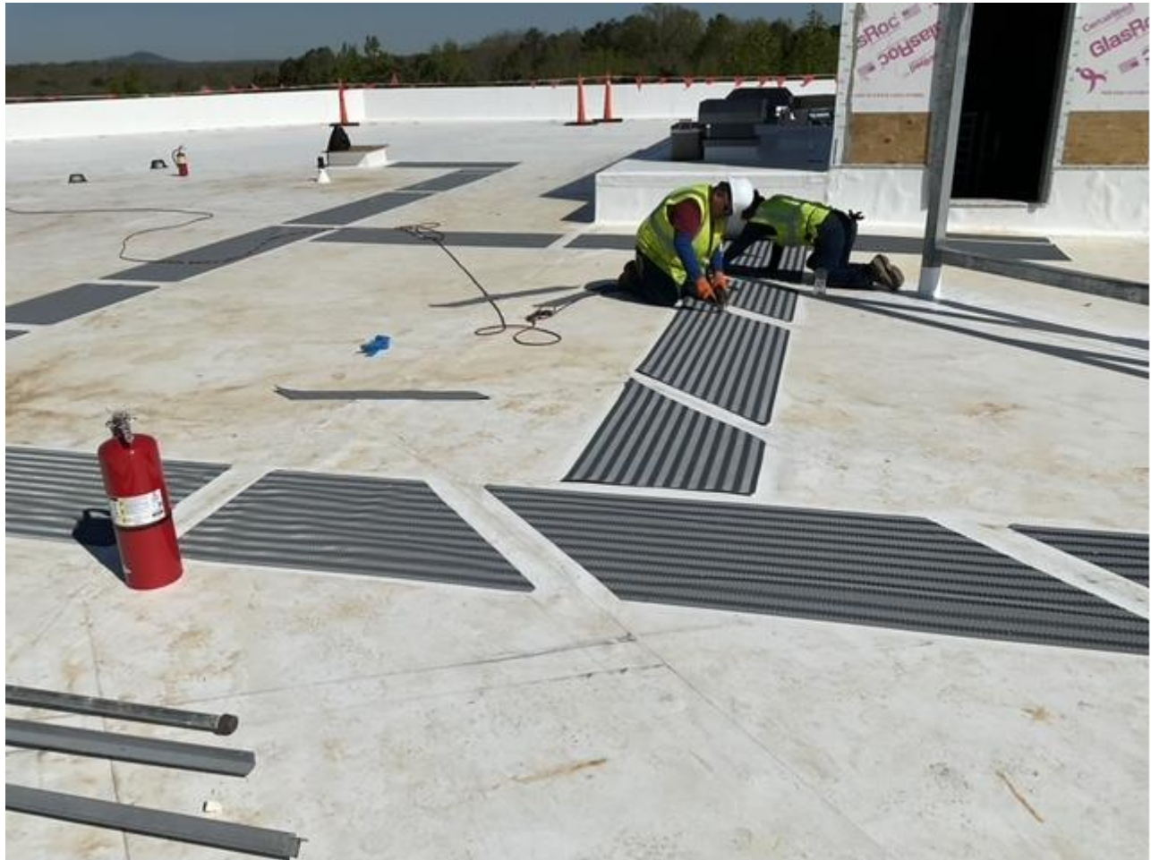
Walks Pads at Roof
