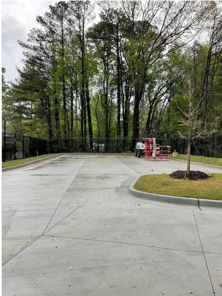
Pressure Washing Concrete Paving
