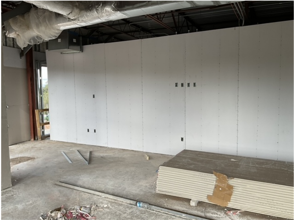
Hanging Drywall on Level 3
