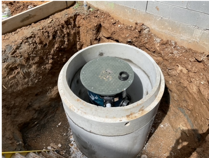
Lift Manhole Station At Sally Port
