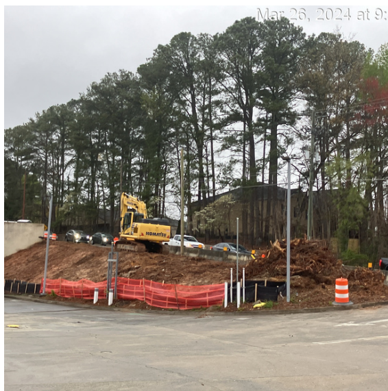
TS191 Grading For New Connector Road
