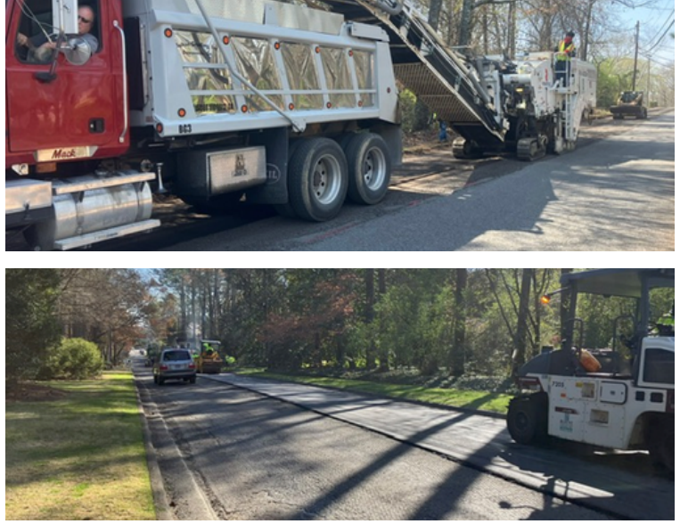
FY24 Resurfacing Project - Jett Ferry Road
