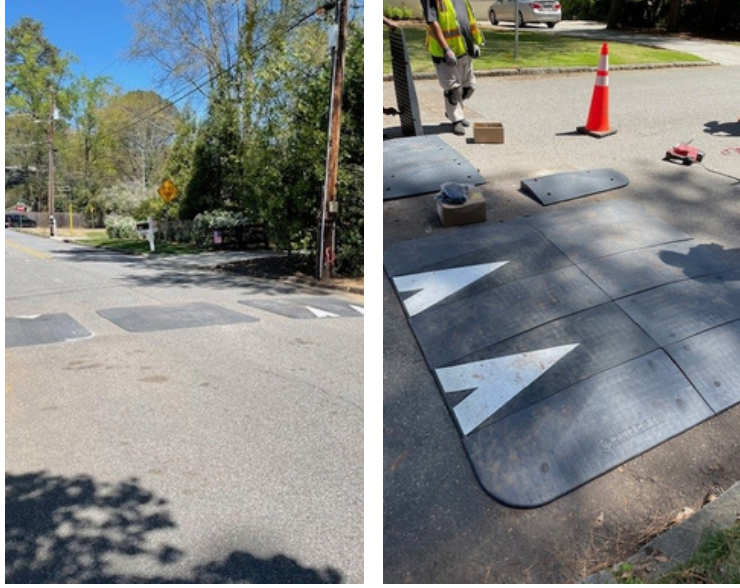
Jolyn Place Speed Cushion Installation
