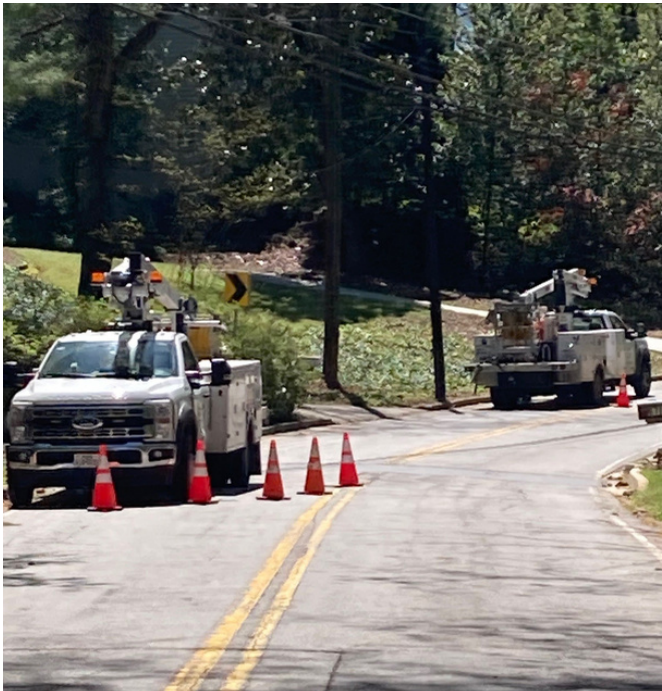
TS172 Brandon Mill Road Sidewalk
