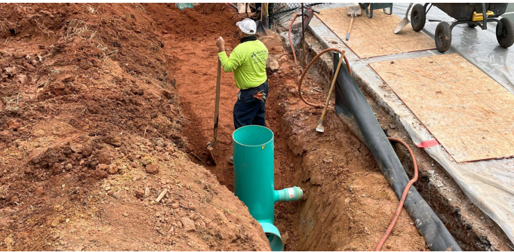
Hammond Park Wall Drainage Installation
