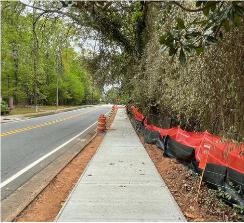
S2170 Mt. Vernon Sidewalk Construction Underway
