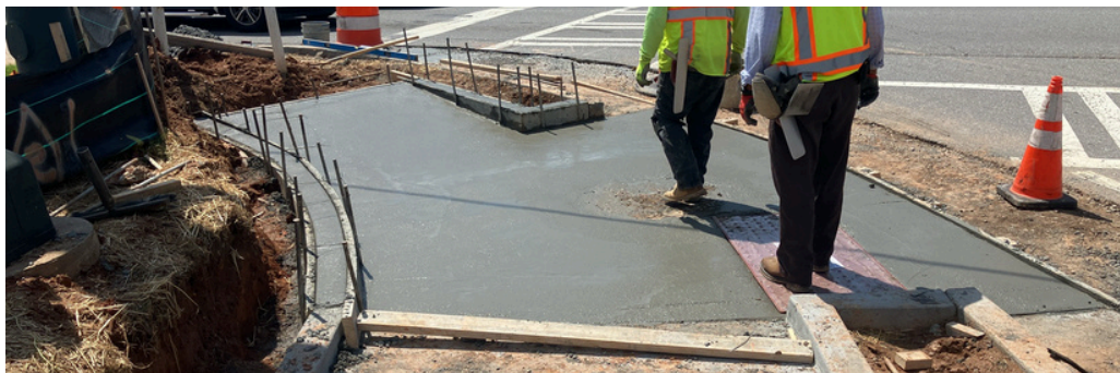
TS108 Sidewalk Ramp Construction
