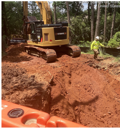
TS191 Storm Drain Installation
