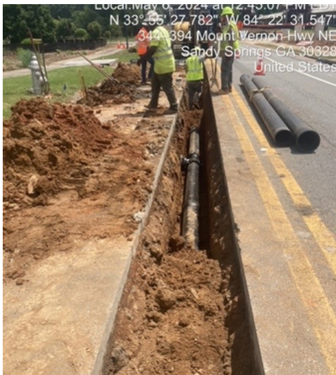
TS191 Waterline Installation
