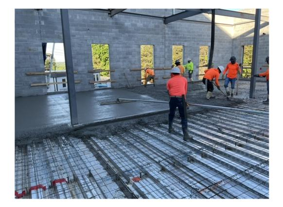
Nelson Studs And Wire Mesh At Elevated Slab
