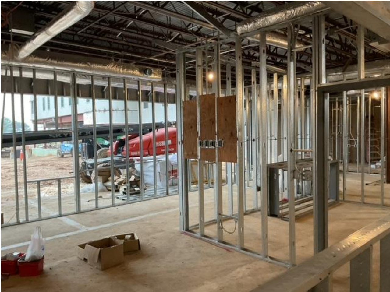
Blocking on 1st floor
