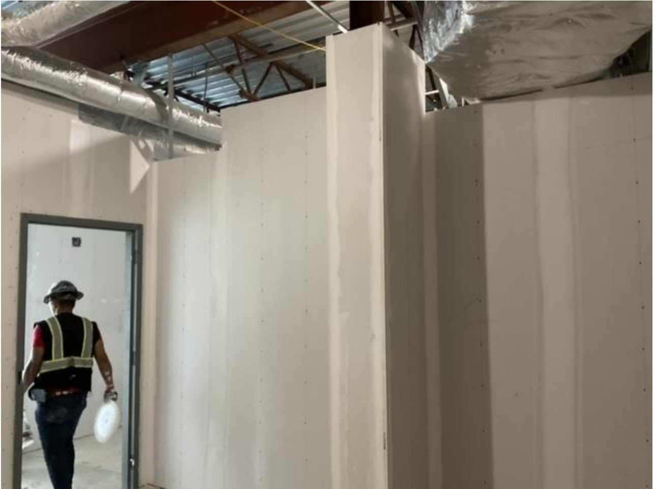
Sheet Rock Finishing
