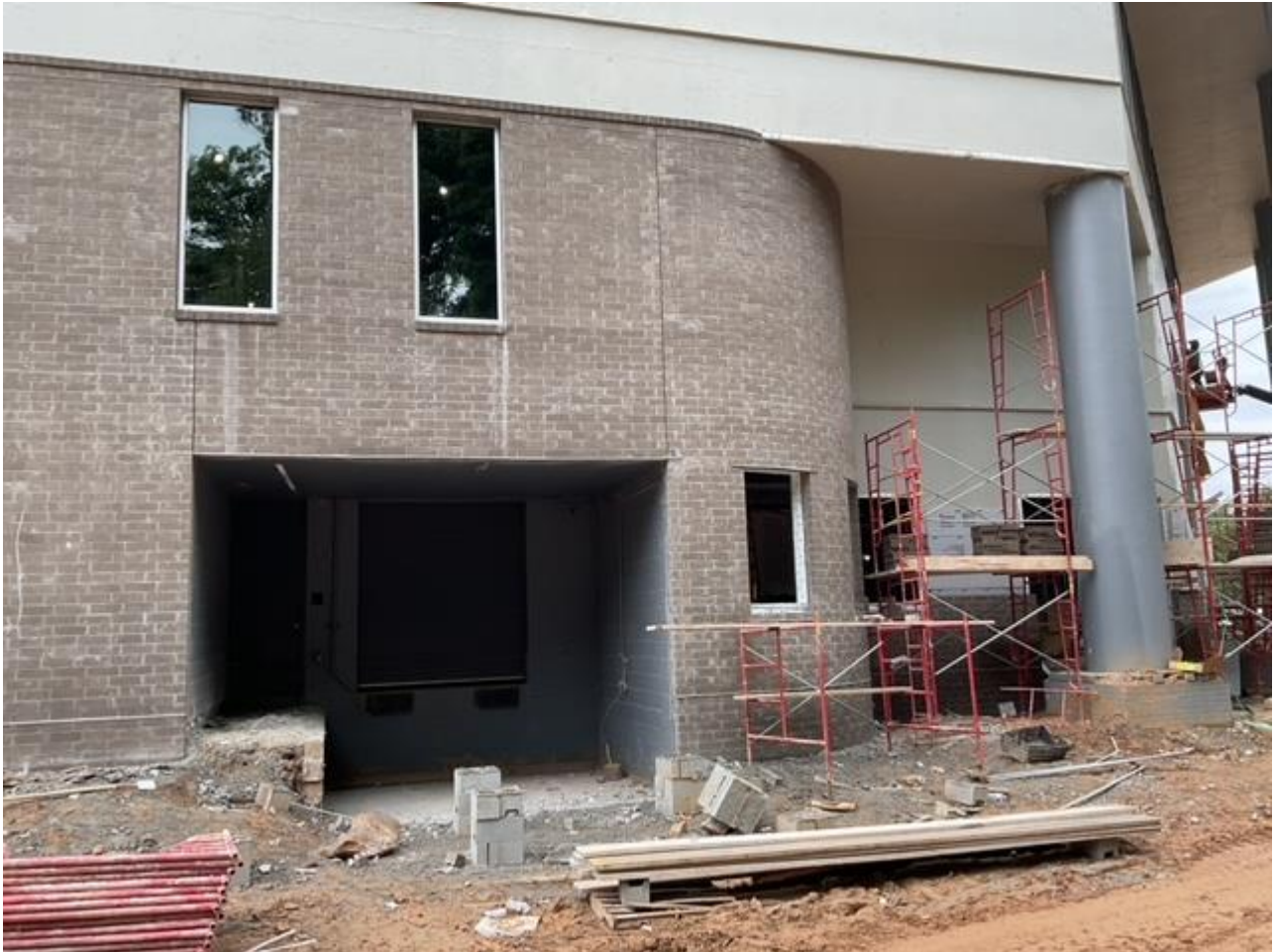
Brick at North Elevation
