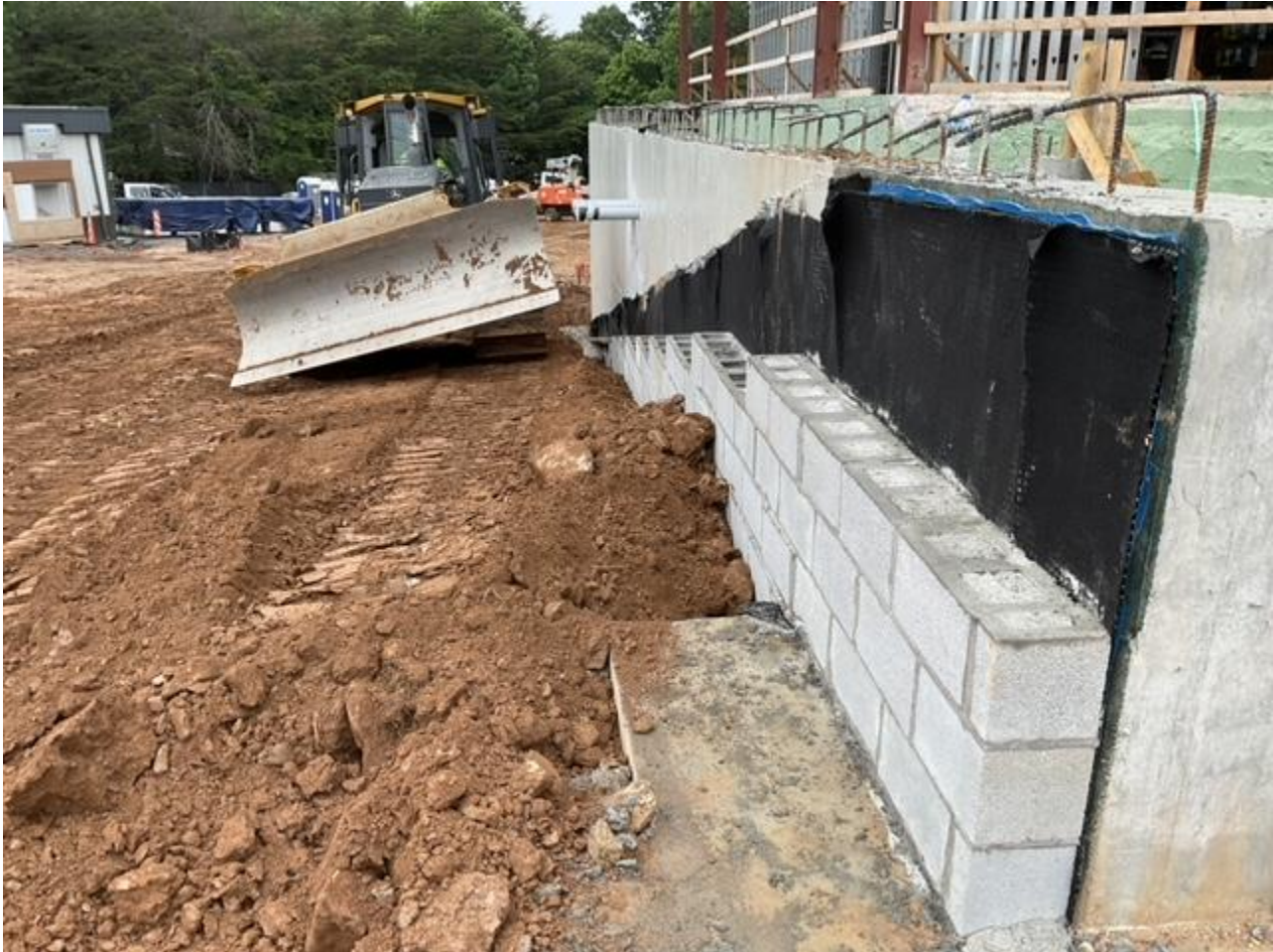
Back fill and block at foundation wall
