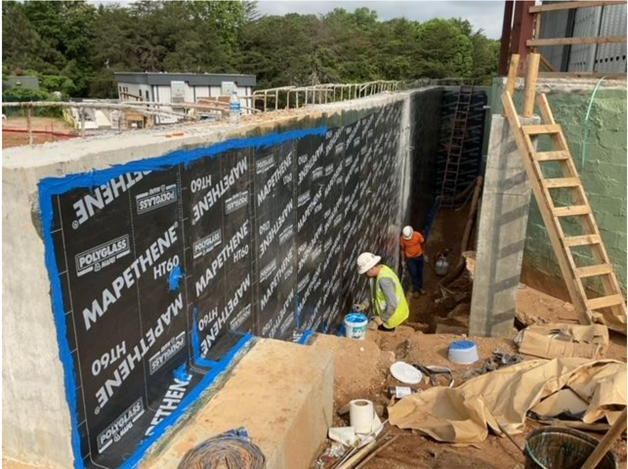
Waterproofing @ Foundation wall
