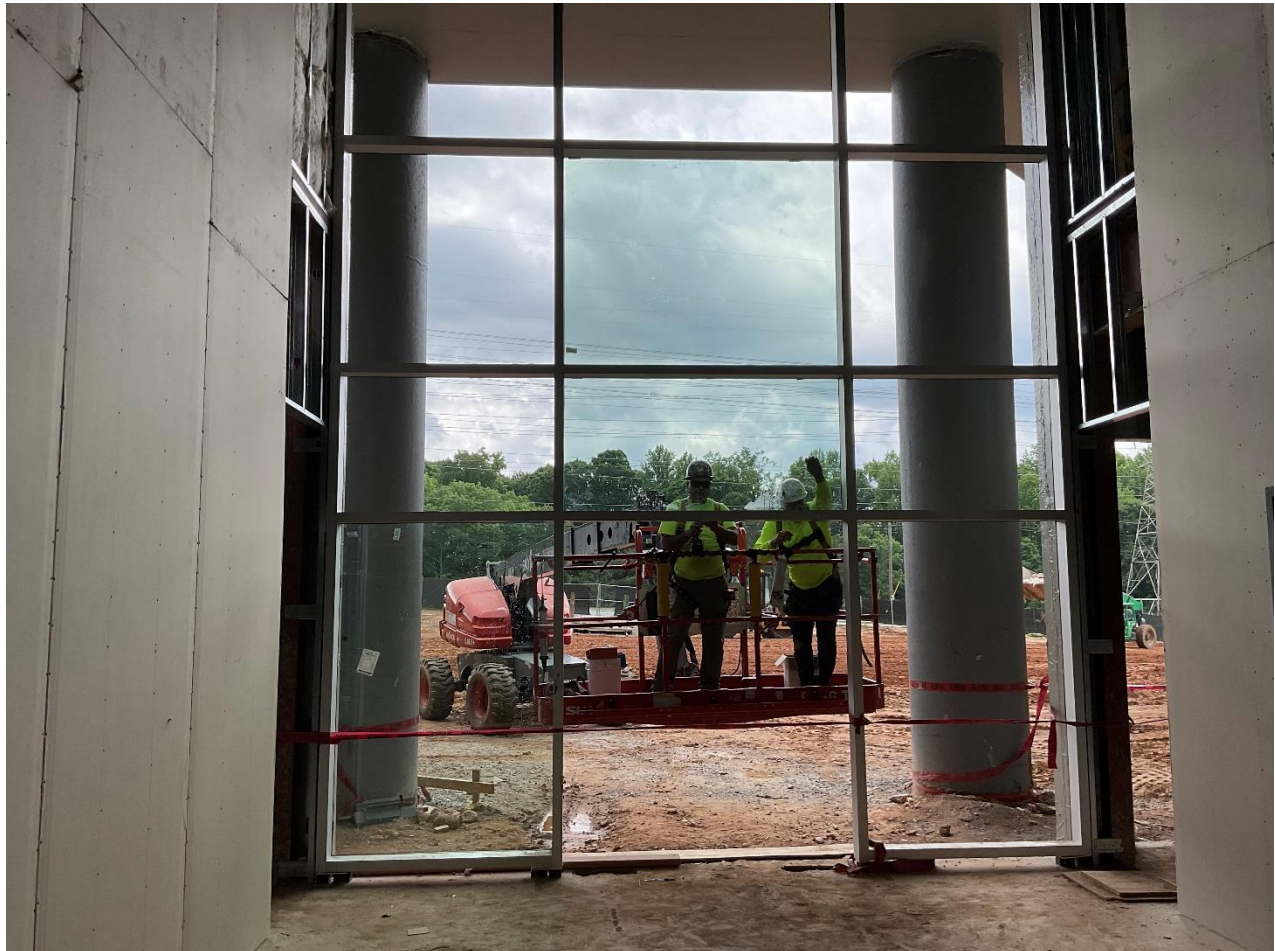
Glazing on 1st floor
