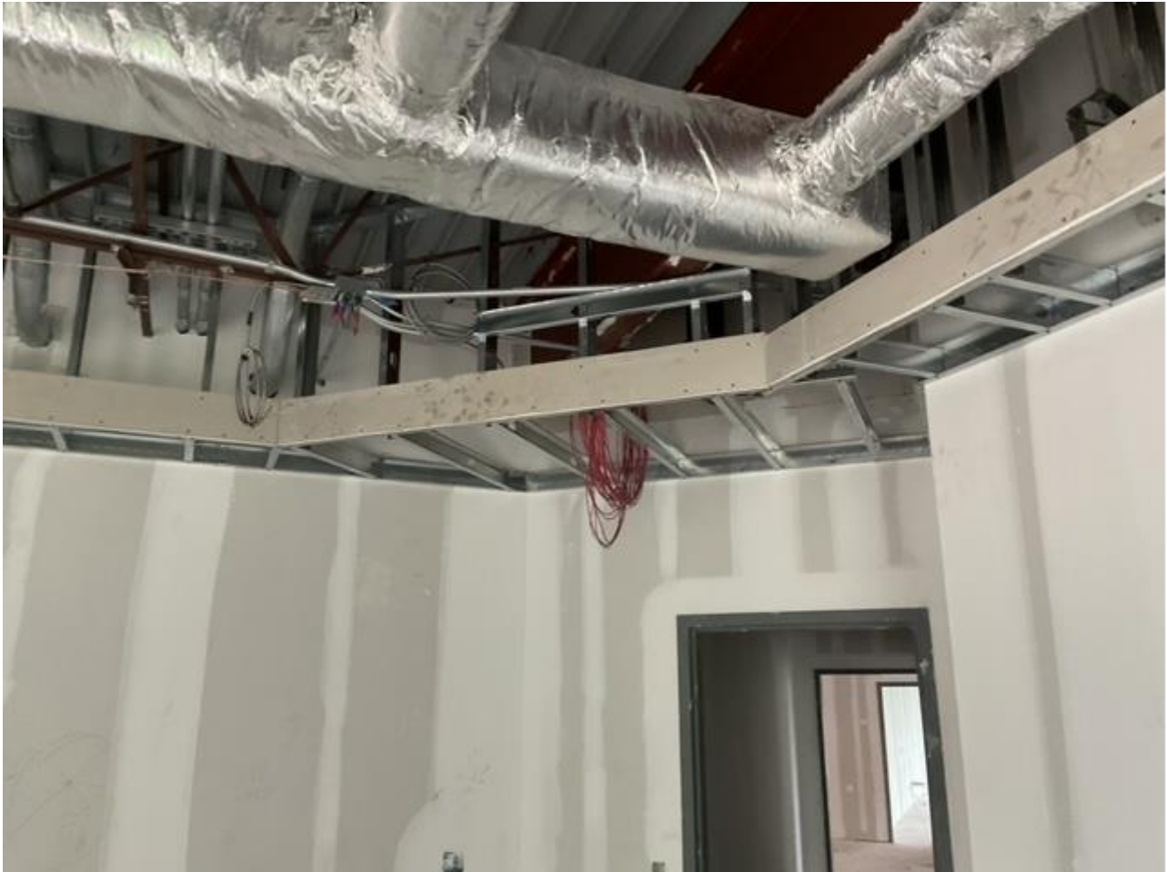
Low Voltage Wire Pulling for Fire Alarm
