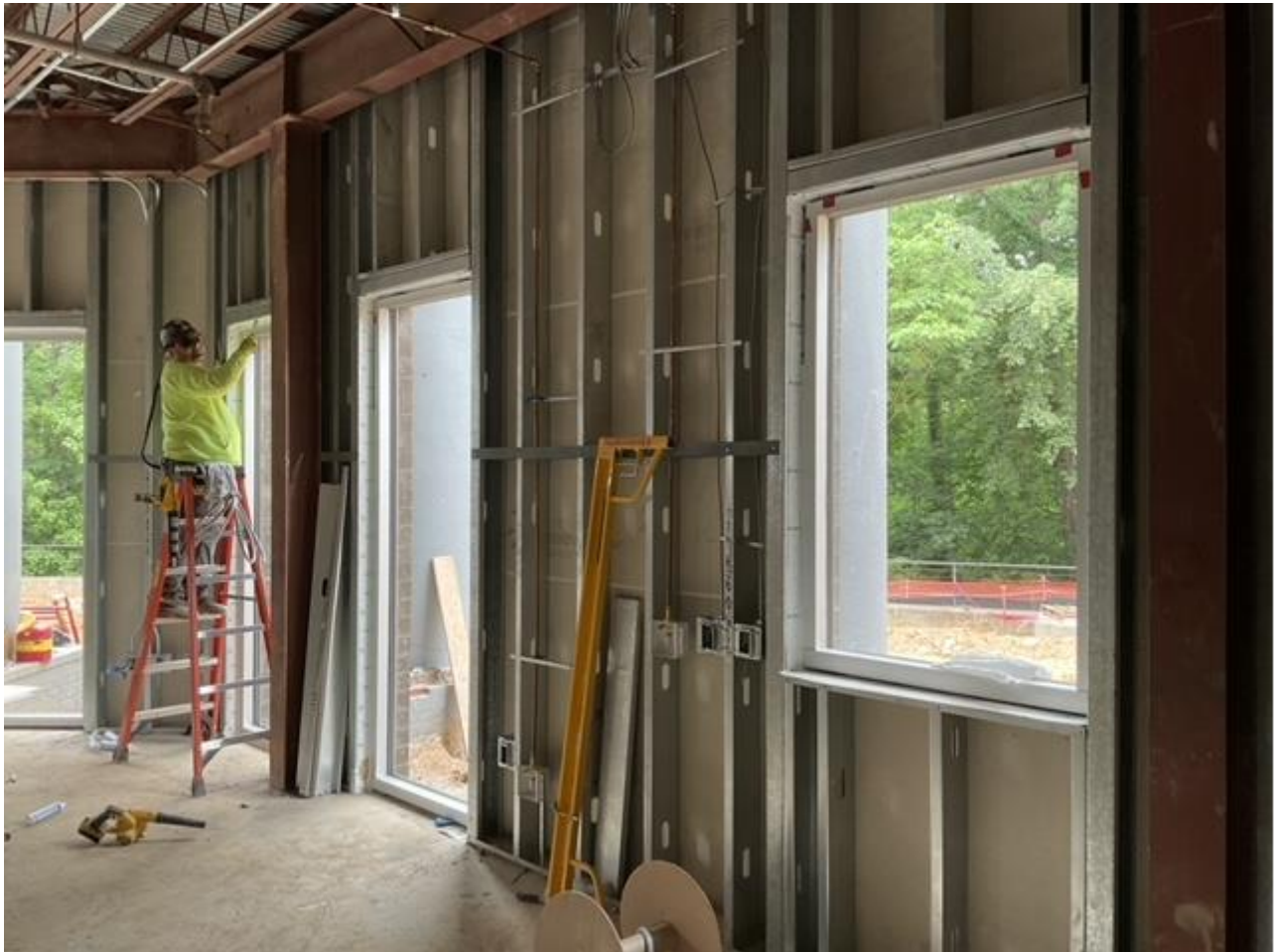
Installing Window Frames
