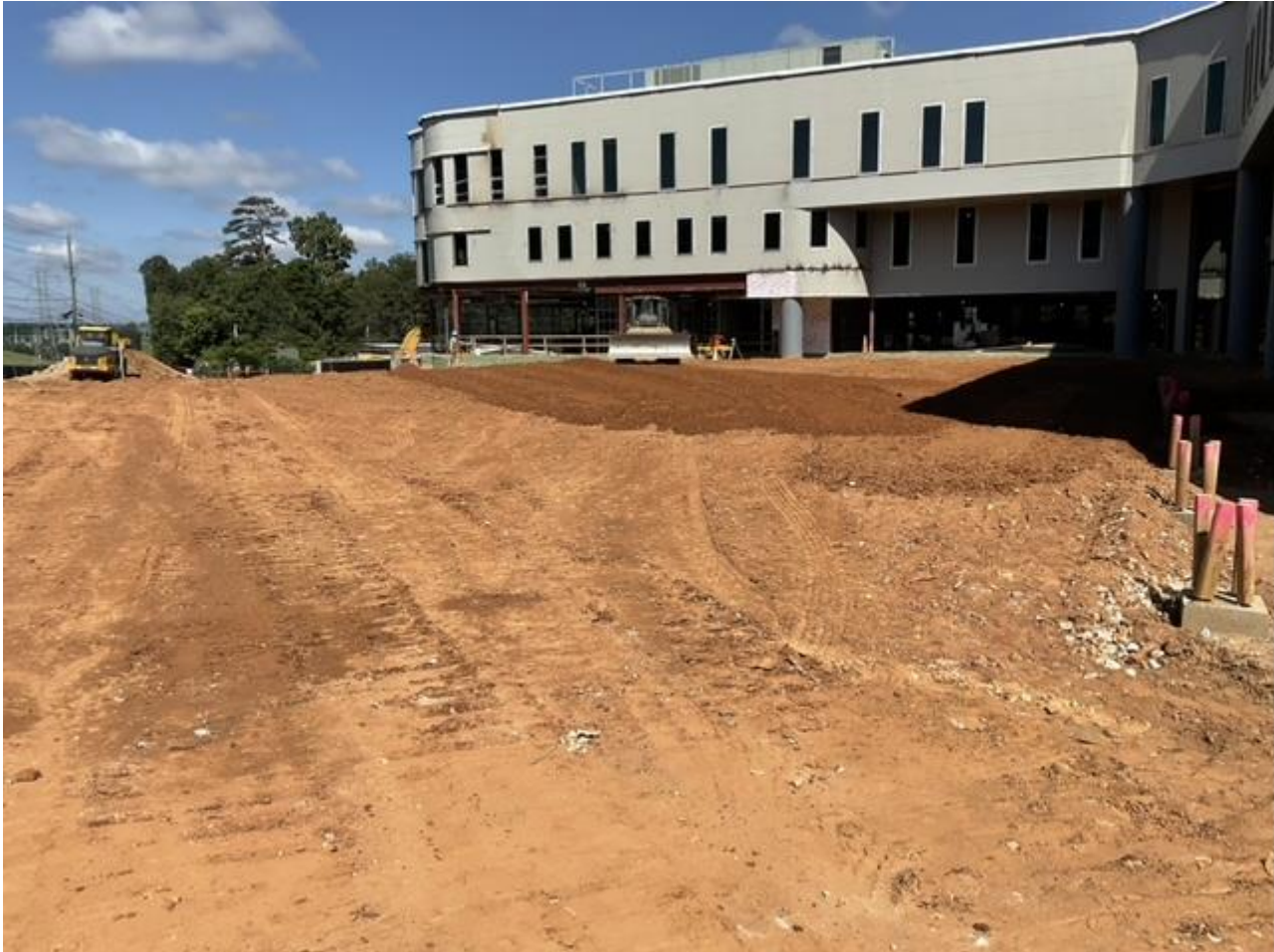
Back Fill at Court House Edition/ Court Yard
