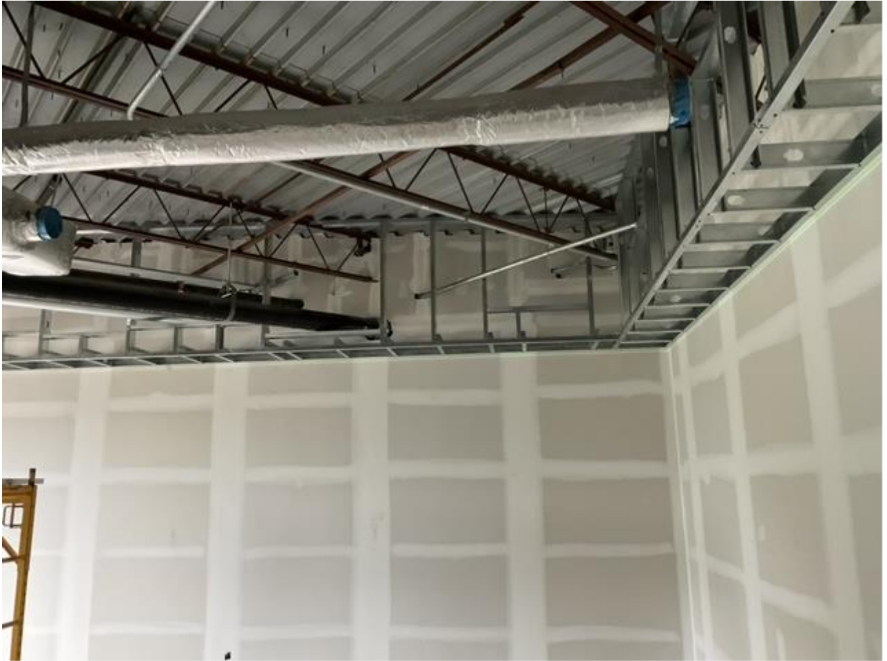
Sheet Rock Finishing
