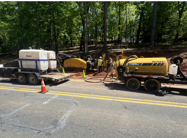
TS111 - Spalding Drive at Pitts Road
