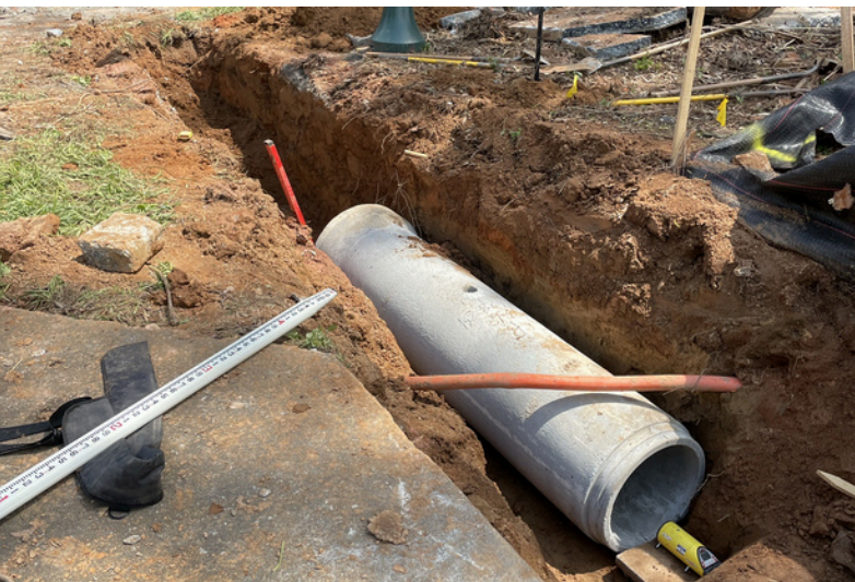
TS191 - Mt. Vernon Highway at Johnson Ferry Road Improvements
