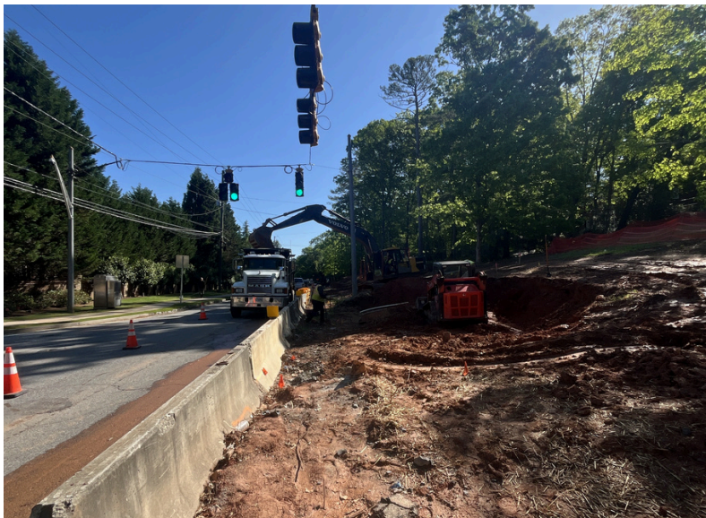
TS111 - Spalding Drive at Pitts Road
