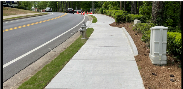
S2175 Trowbridge Sidewalk Construction Completed
