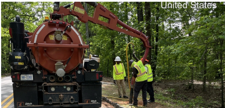
S2165 Riverside Drive Sidewalk Utility Locate Investigation
