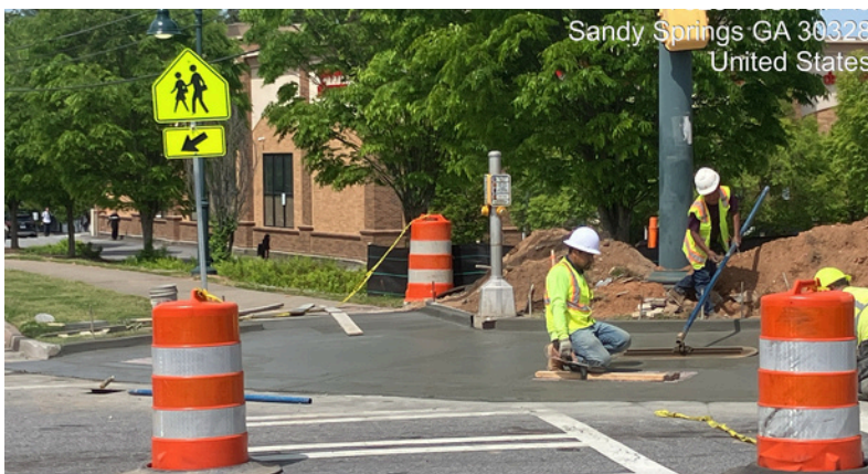
TS108 Sidewalk Installation
