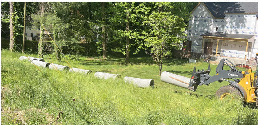
TS111 Storm Drain Installation
