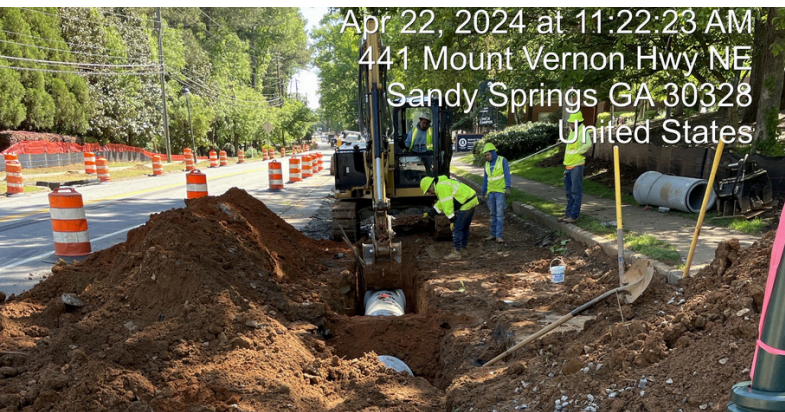
TS191 Storm Drain Installation
