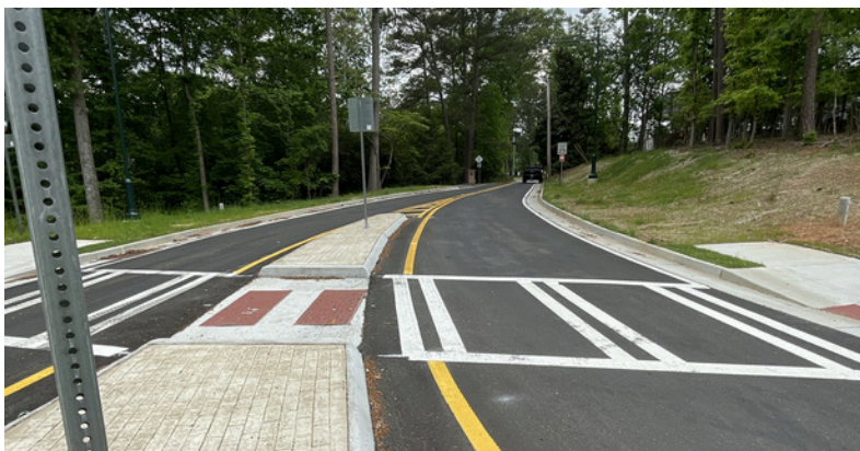
TS106 Final Striping
