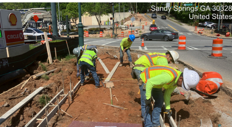
TS108 Curb and Gutter Installation
