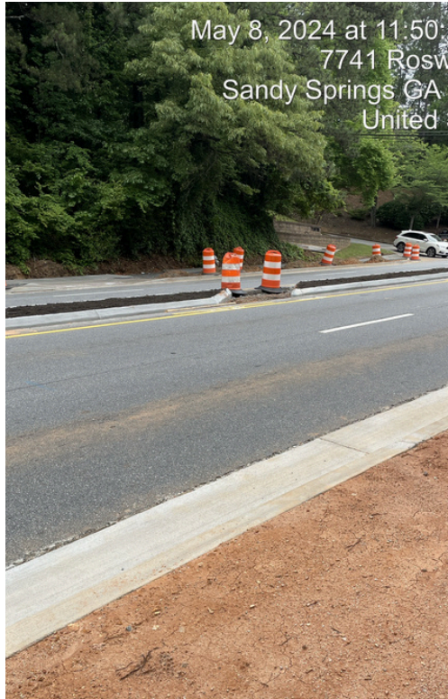
T2205 Mid-block Crossing Median Work
