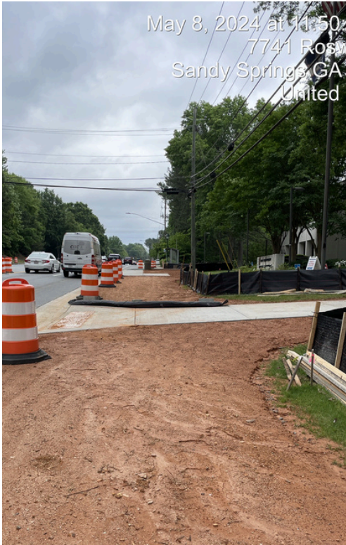
T2205 Mid-block Crossing Shoulder Work
