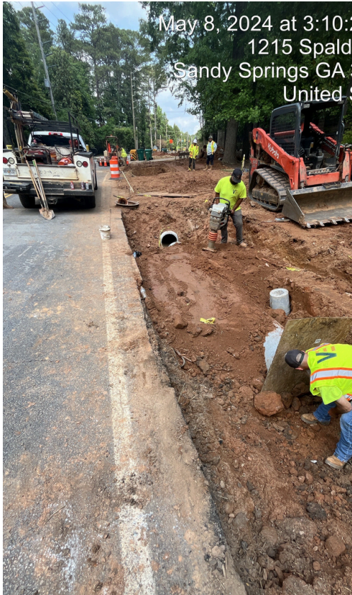
TS111 Storm Drain Installation
