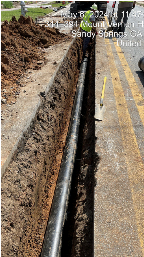
TS191 Waterline Relocation
