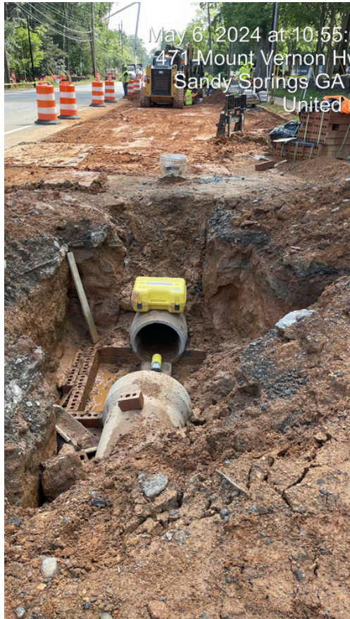
TS191 Storm Drain Installation
