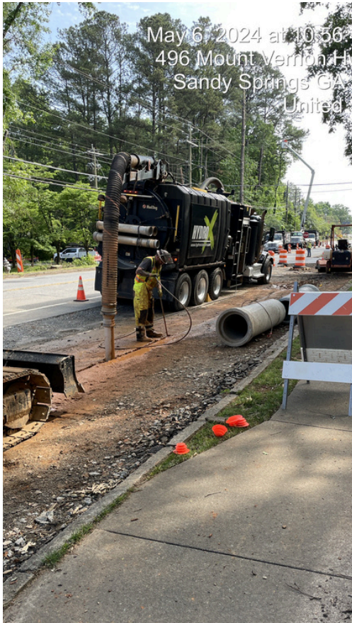
TS191 Storm Drain Installation
