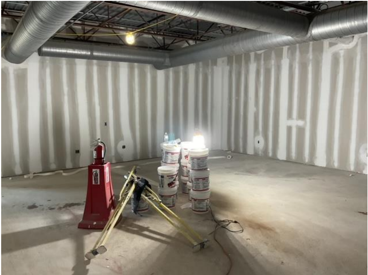
Sheet Rock Finishing
