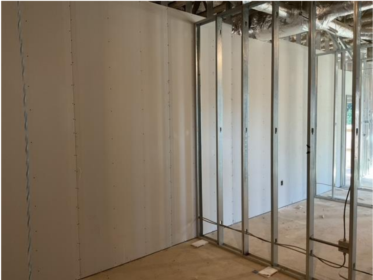
Instillation of Sheet Rock on 1 st Floor
