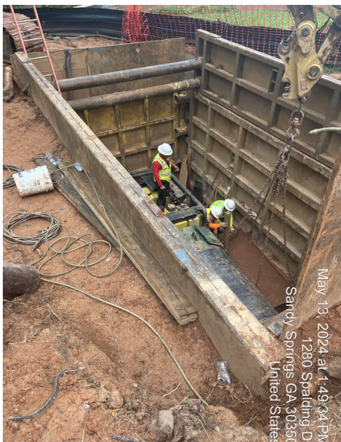
TS111 Storm Drain Installation
