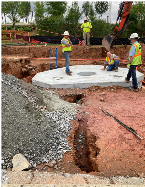
TS191 Underground Utility Vault Installation
