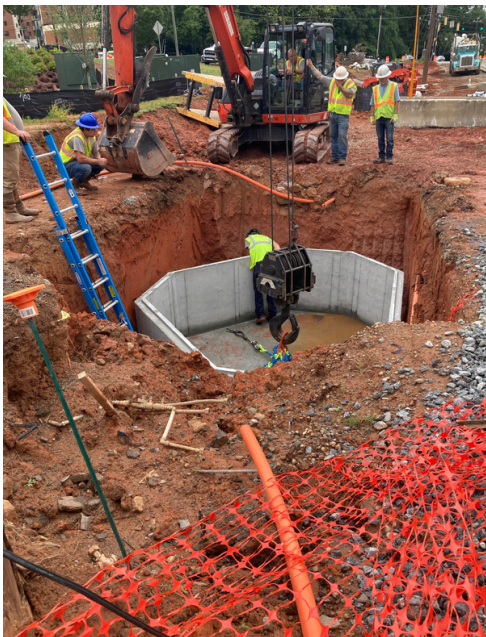
TS191 Underground Utility Vault Installation
