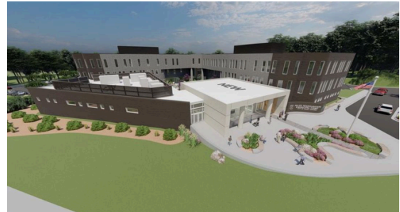
POLICE HEADQUARTERS AND COURT
