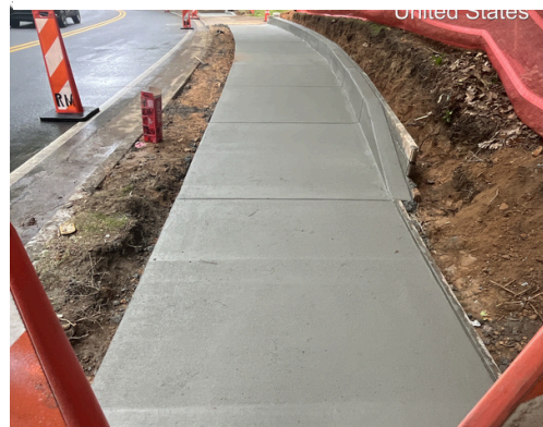
S2188-4 Sidewalk Construction
