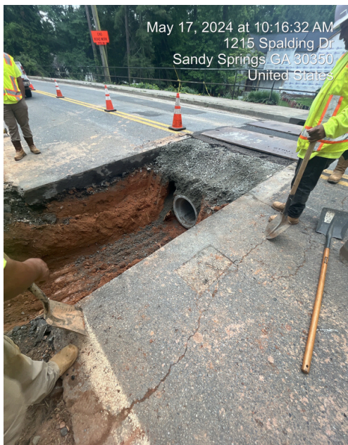
TS111 Storm Drain Installation
