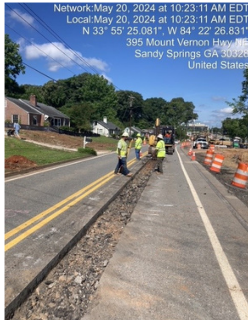
TS191 Waterline Relocation
