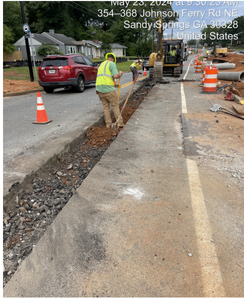
TS191 Stormwater System Construction
