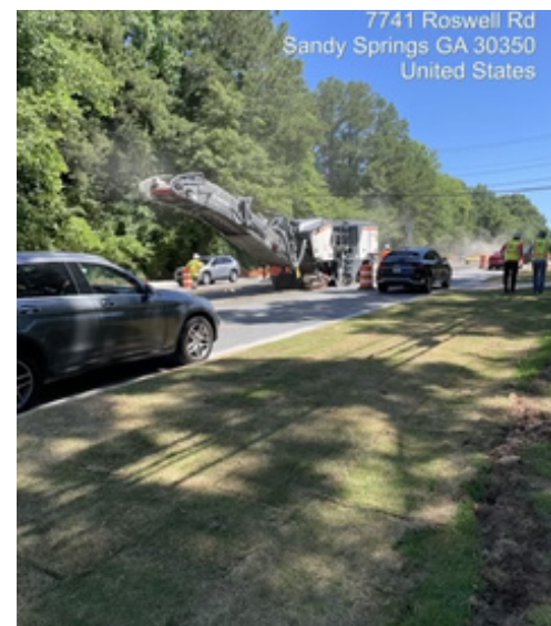
T2205-01 Mid-block Crossing Roadway Milling
