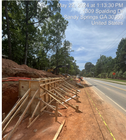
TS111 Retaining Wall Construction
