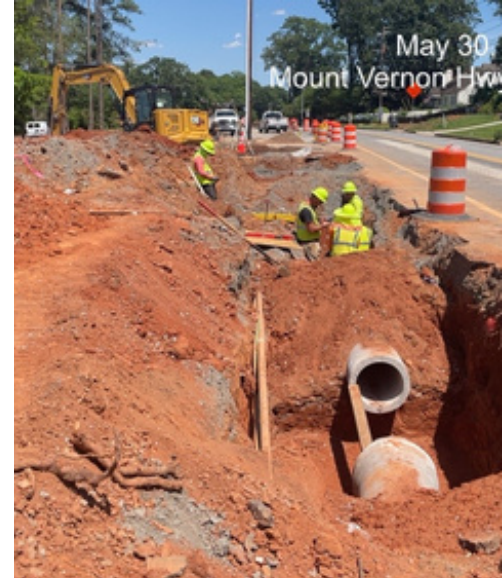
TS191 Storm drain installation Mt. Vernon Hwy
