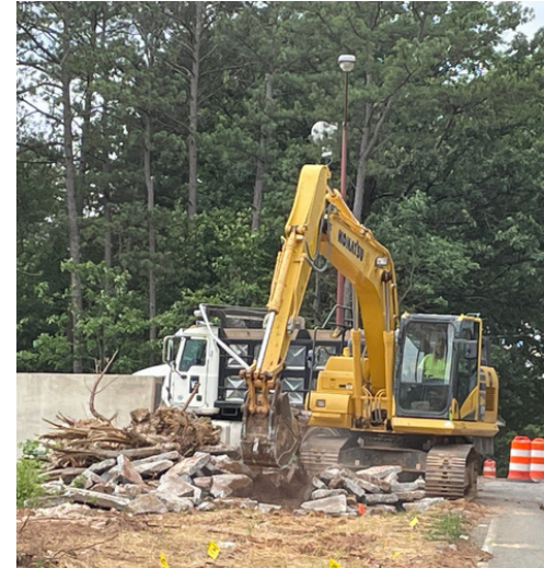
TS108 Sidewalk demolition and wall preparation
