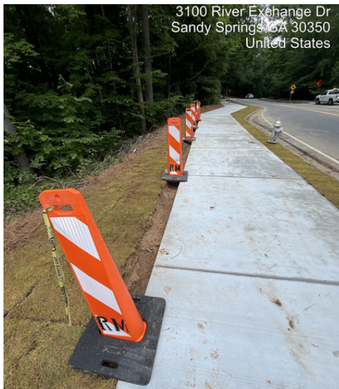
S2188-5 Windsor Parkway Sidewalk construction
