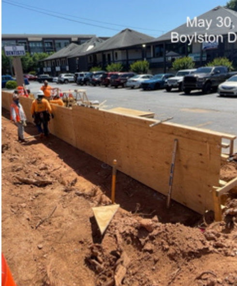
TS191 Wall construction Boylston Drive
