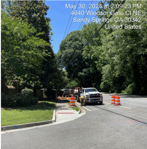
T0069 Peachtree Dunwoody - Windsor Pkwy Traffic Fiber Connection underground boring
