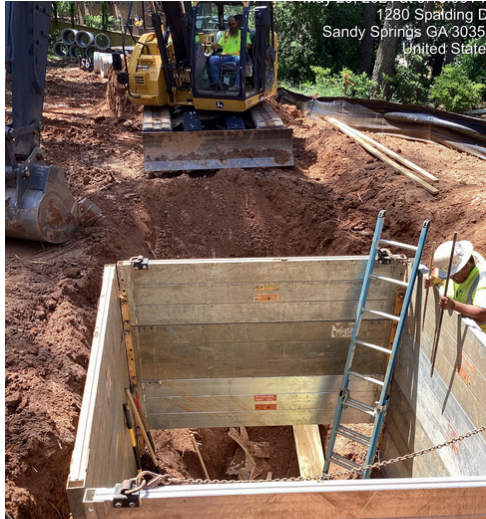
TS111 Stormwater System Construction
