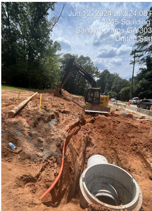
TS111 Stormwater Installation
