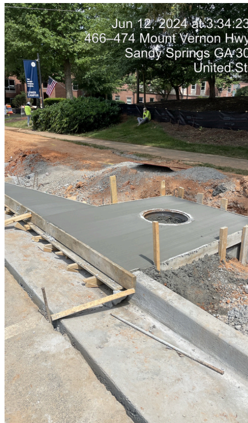
TS191 Storm Inlet Construction Mt. Vernon Highway
