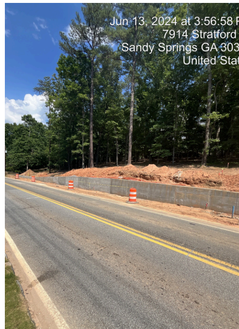
TS111 Retaining Wall Construction
