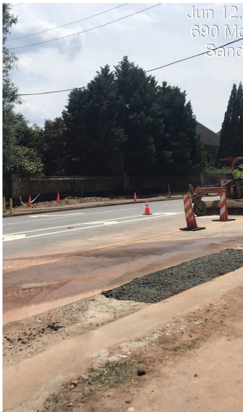
TS192 Water Line Installation Roadway Repairs Mt. Vernon Highway
