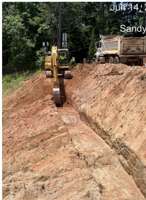
TS108 Retaining Wall Construction
