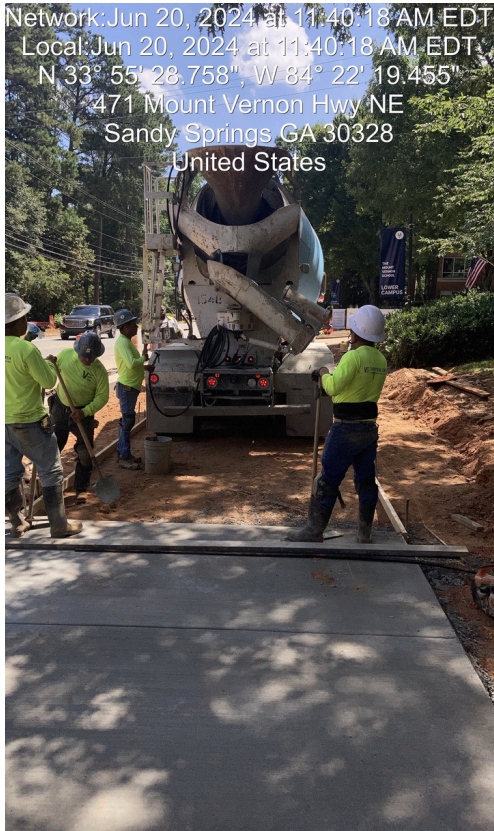
TS191 Mt Vernon Multi-use Path Construction
