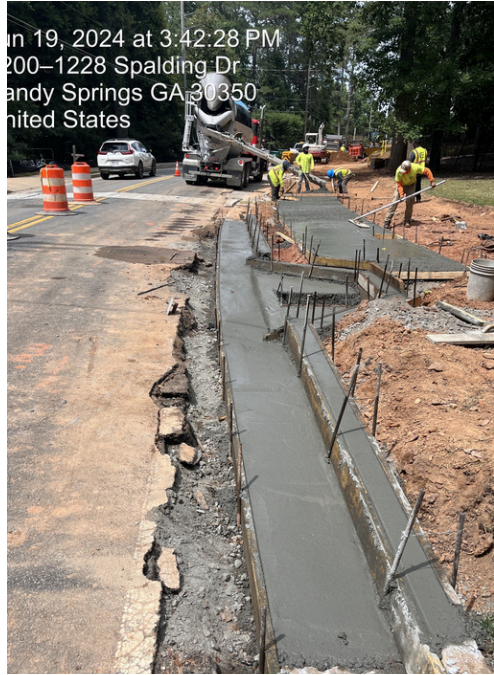
TS111 Curb and Gutter and Sidewalk Construction
