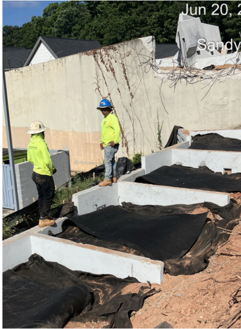
TS108 Wall Installation
