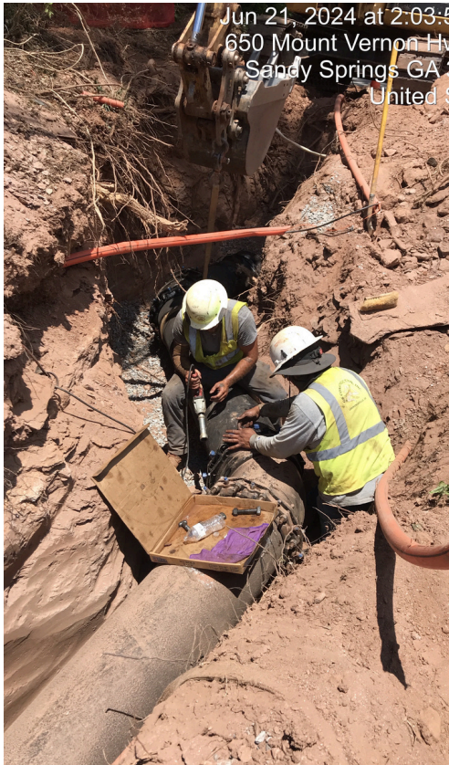
TS191 Waterline Relocation
