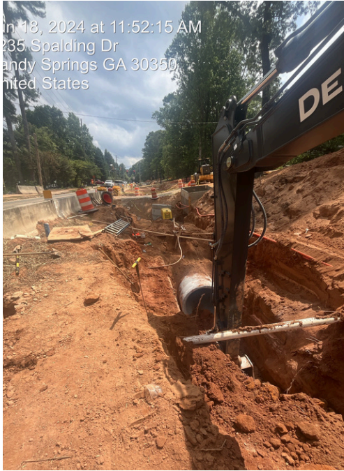
TS111 Stormwater Construction
