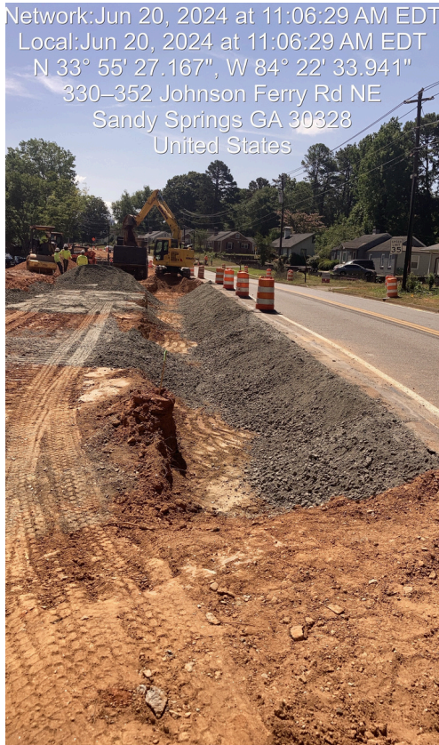
TS191 Johnson Ferry Roadway Construction
