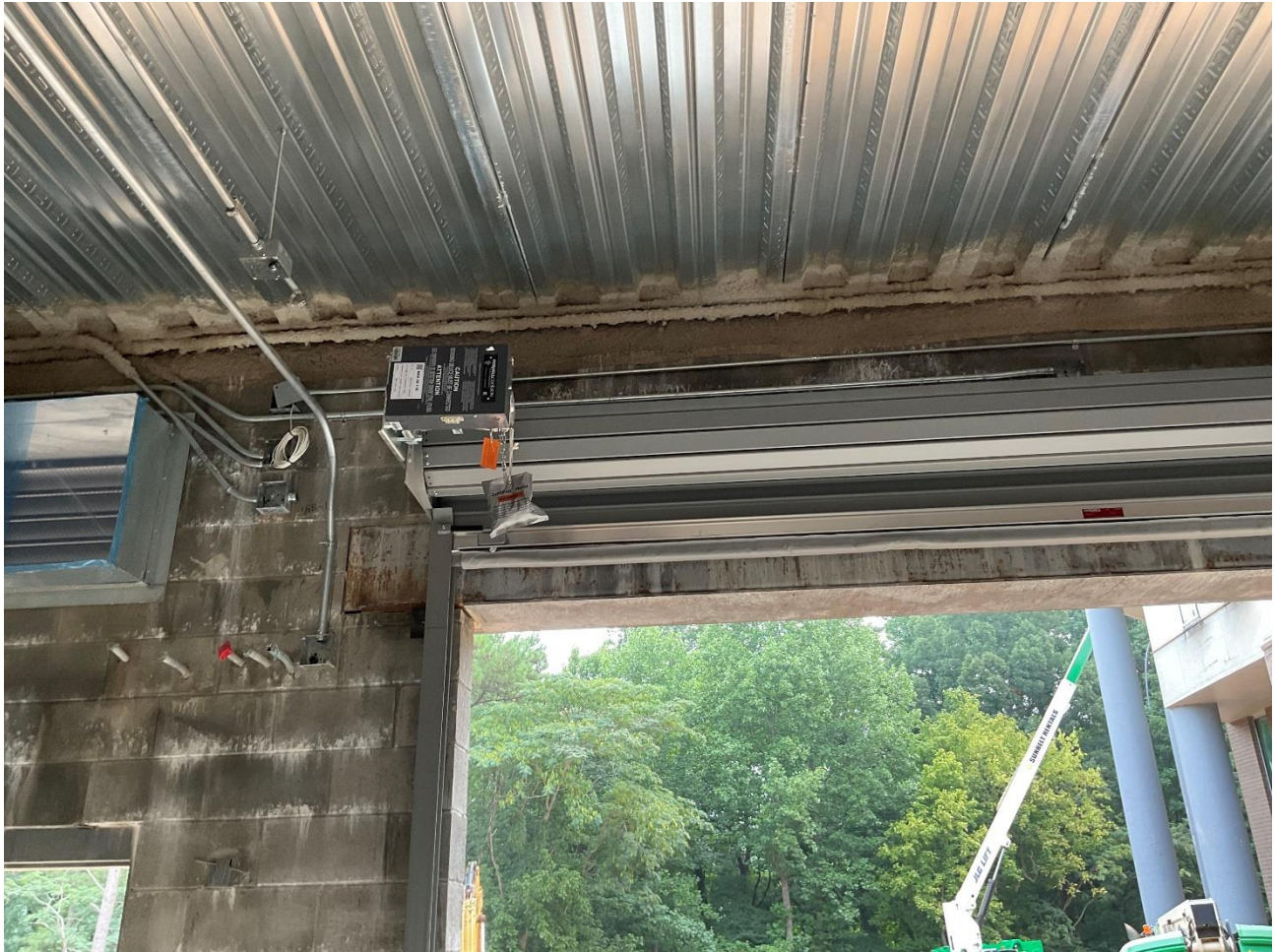
O/H Door Install @ Sally Port
