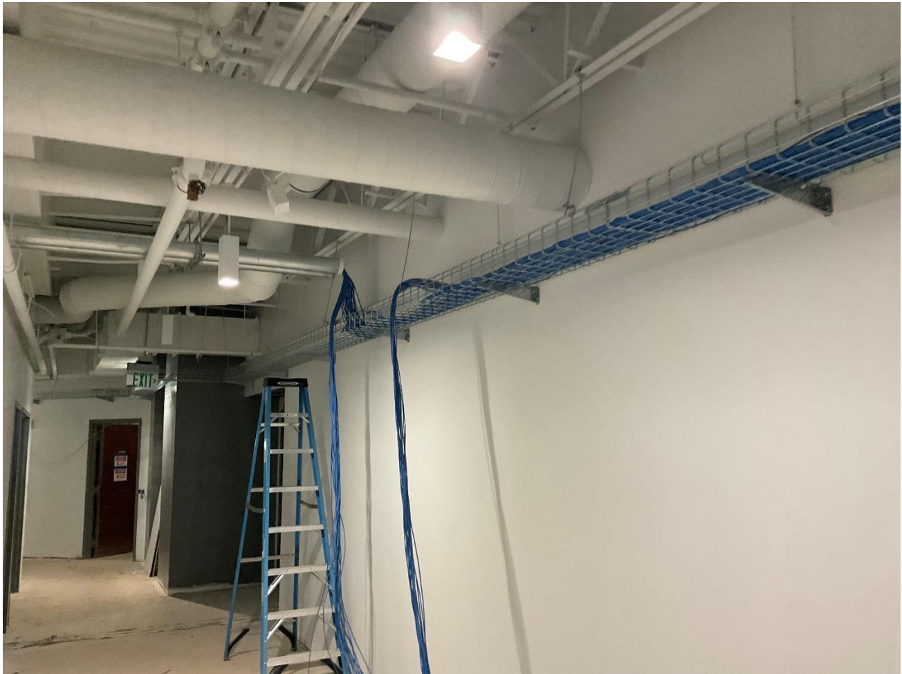
Pulling LV Cables
