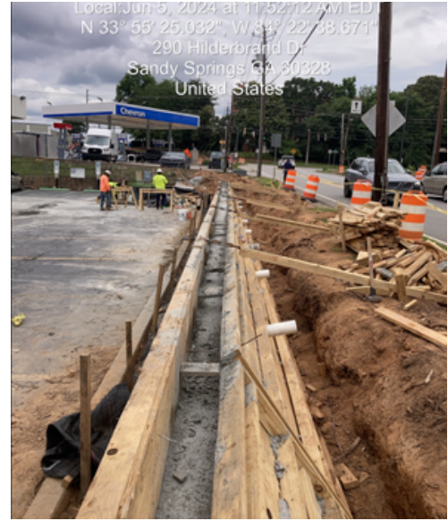
TS191 Stormwater Installation
