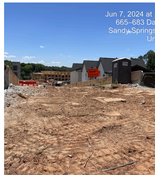
TS108 Wall Preparation
