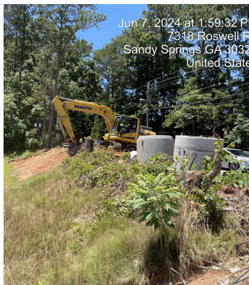
TS108 Wall Preparation
