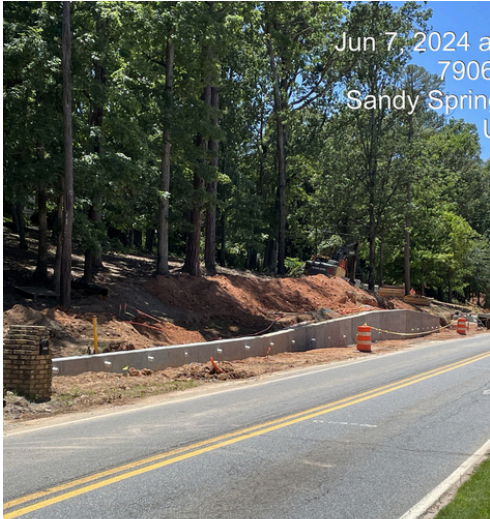
TS111 Wall Construction
