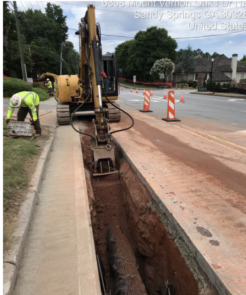
TS192 Waterline Installation
