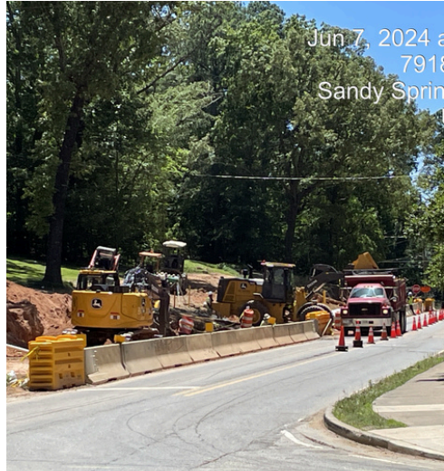
TS111 Stormwater Installation
