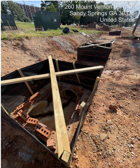
TS191 Wall Construction
