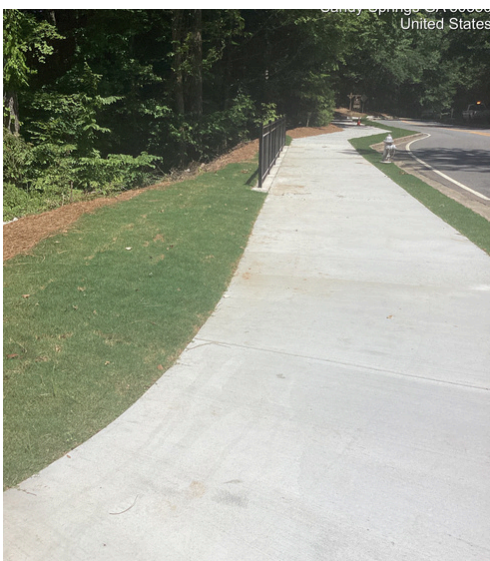
S2188-4 River Exchange Sidewalk Completed
