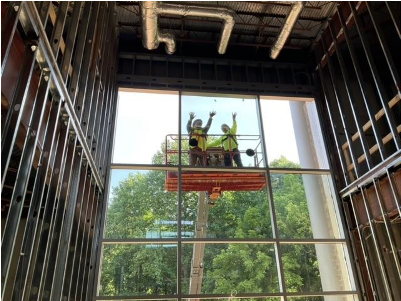
Glazing Install @ basement
