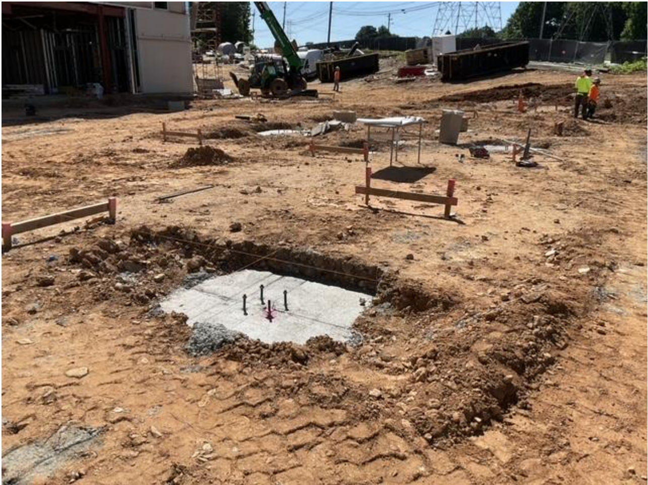
F/R/P footings @ Courtroom
