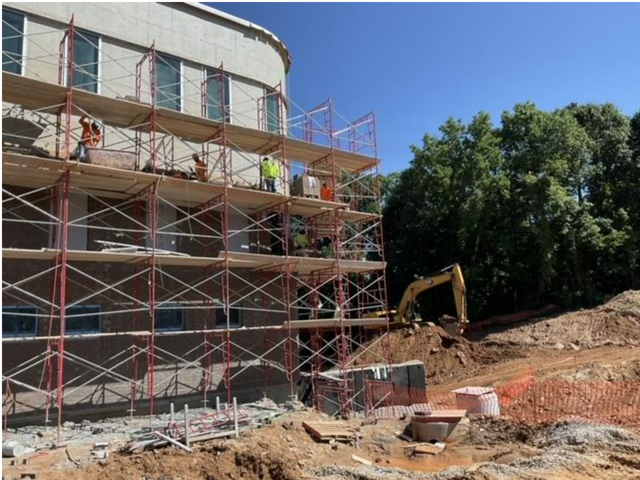
Brick install @ North radius
