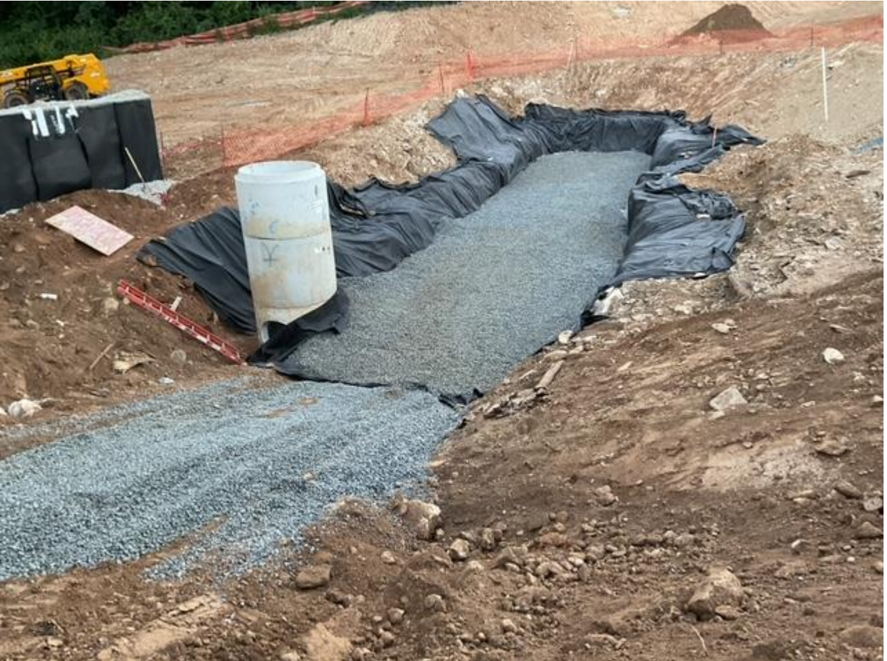
Excavate/install Bio cell
