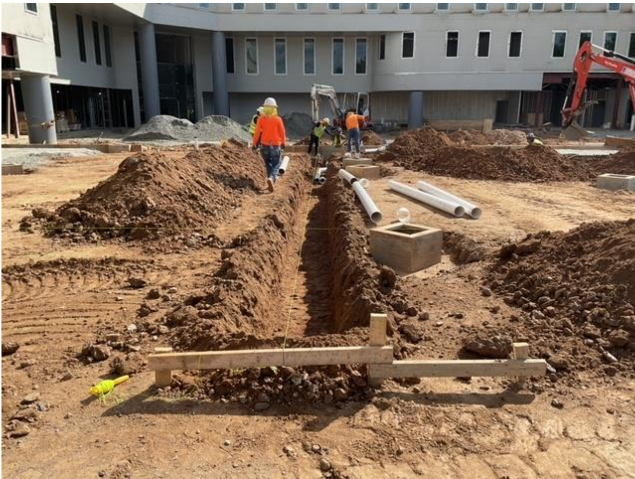
Underground plumbing rough in
