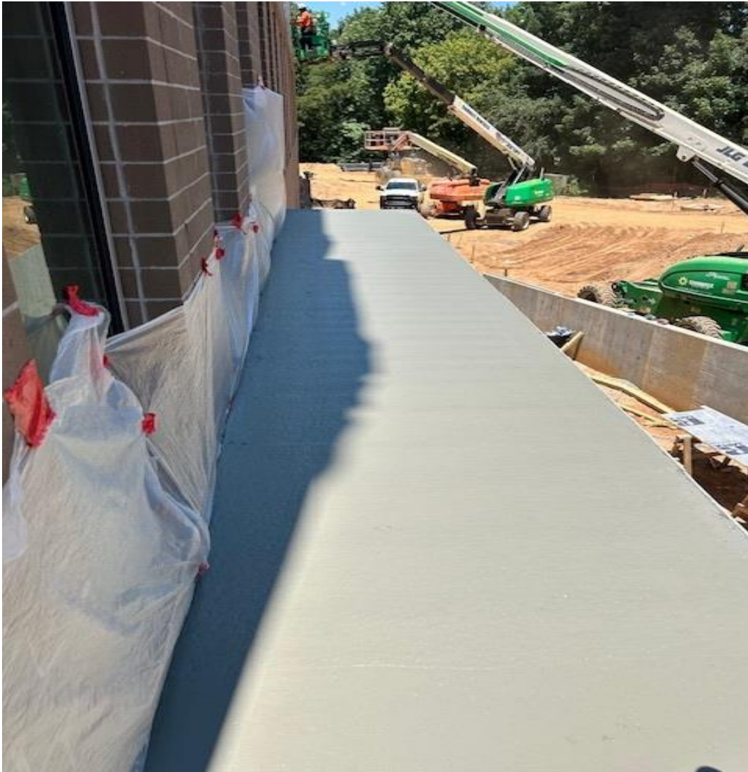
Pouring of Elevated sidewalk
