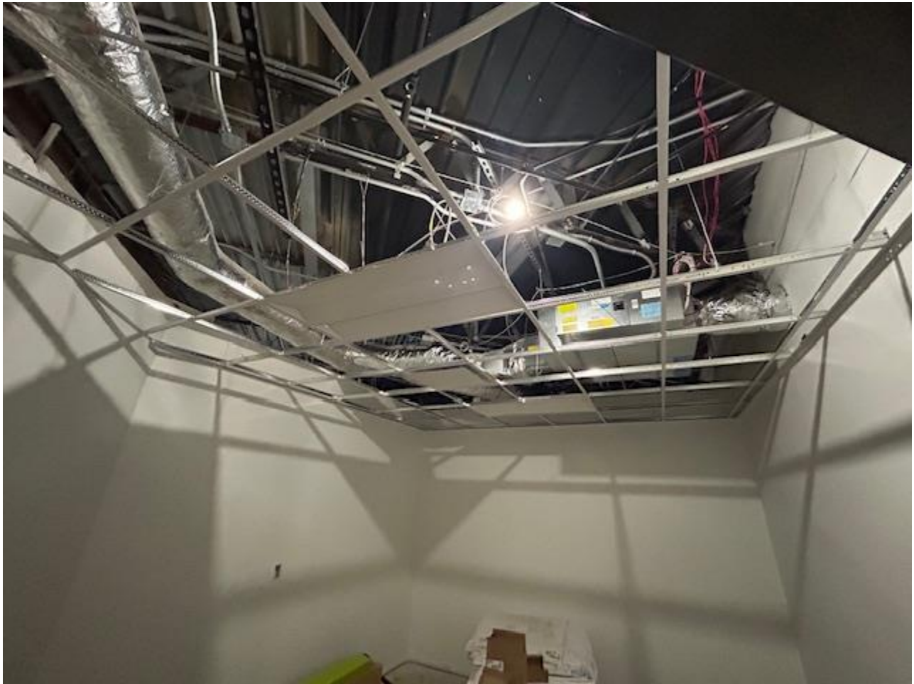
Diffuser and light install
