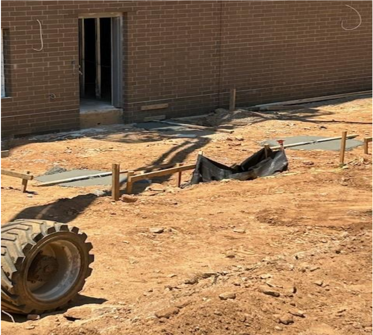
Pouring of canopy footings
