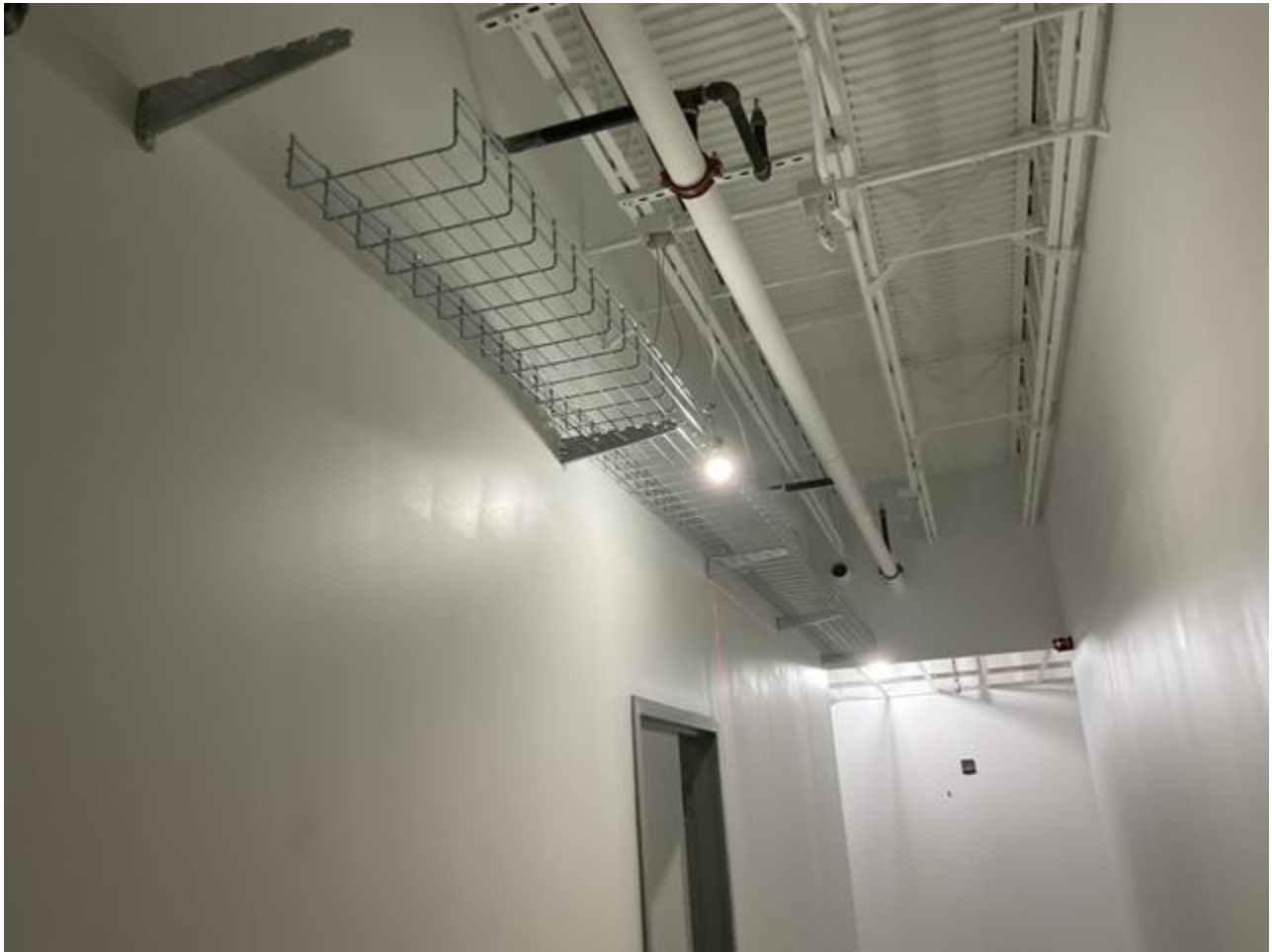
Cable Tray install
