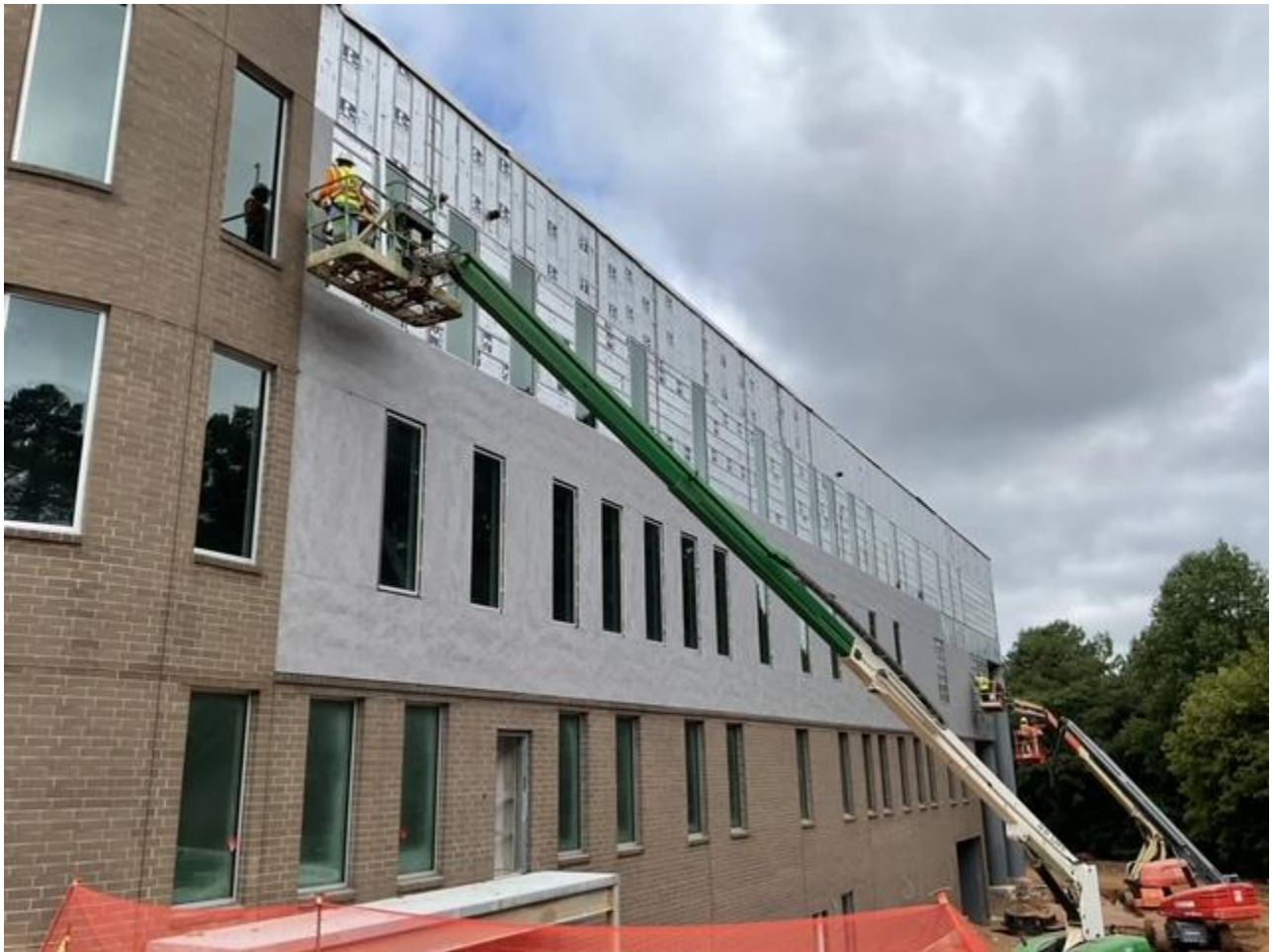
Fiber cement siding install
