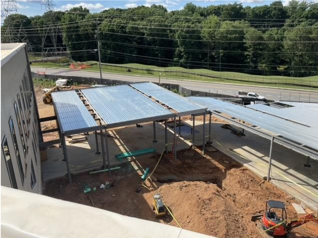
Roof Decking Install
