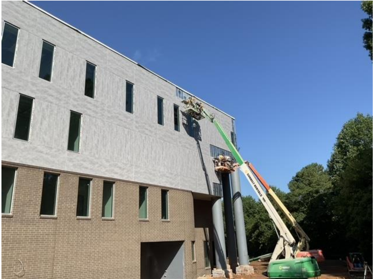
Fiber cement siding install
