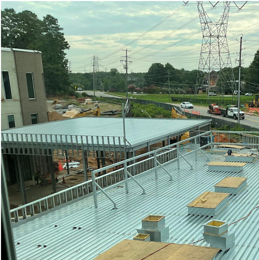
Parapet Framing, Screenwall Steel & Roof Curbs at Addition B
