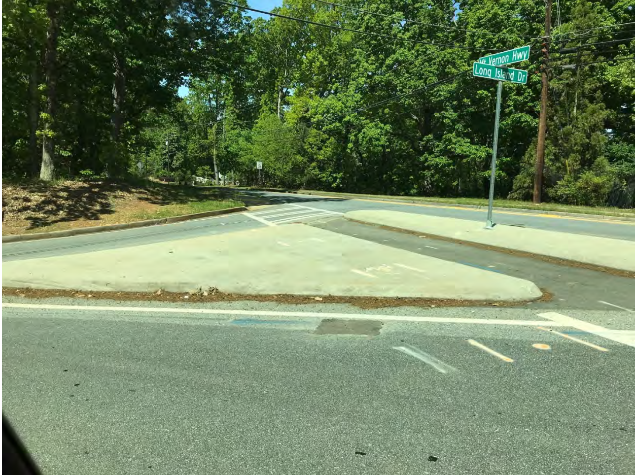
Figure 9: View from the Long Island Drive left turn with front of vehicle at the stop bar. Note how embankment and a few trees still block adequate (390') sight distance. Suggest crews do additional clearing.
