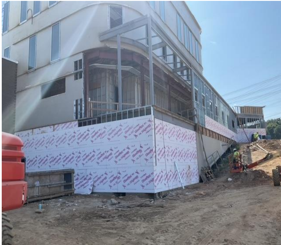
Sheathing at Swat Room
