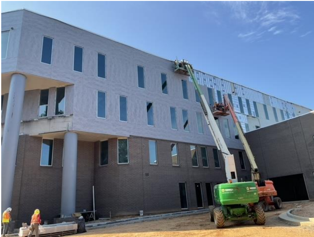
Fiber-Cement Siding at West Elevation
