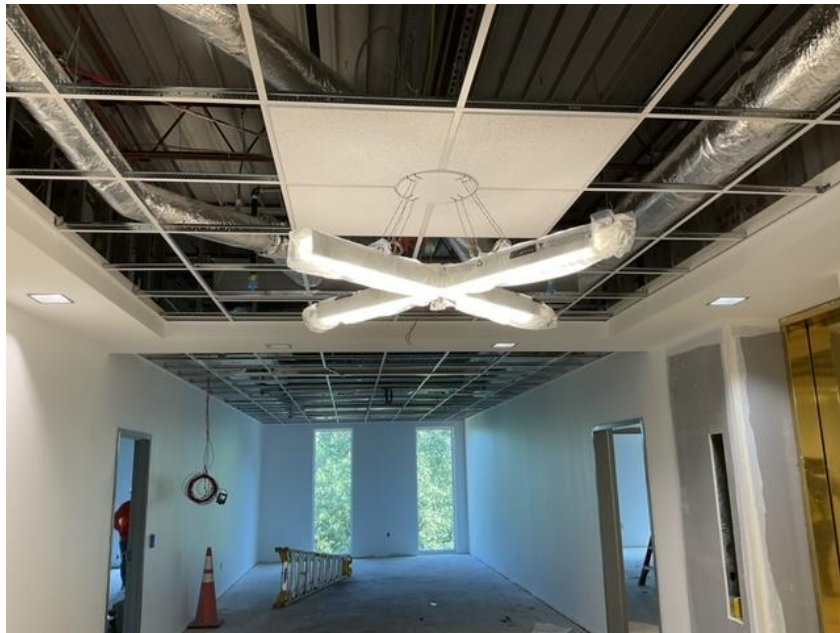
Light Fixture at 3 rd Floor Corridor
