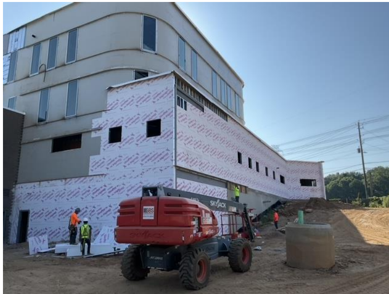
Sheathing @ Corner of North & South Elevations
