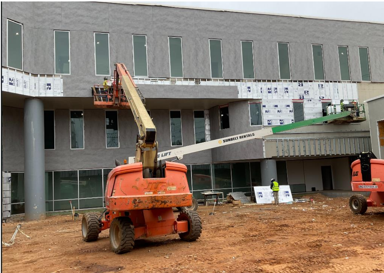
Siding at Courtyard
