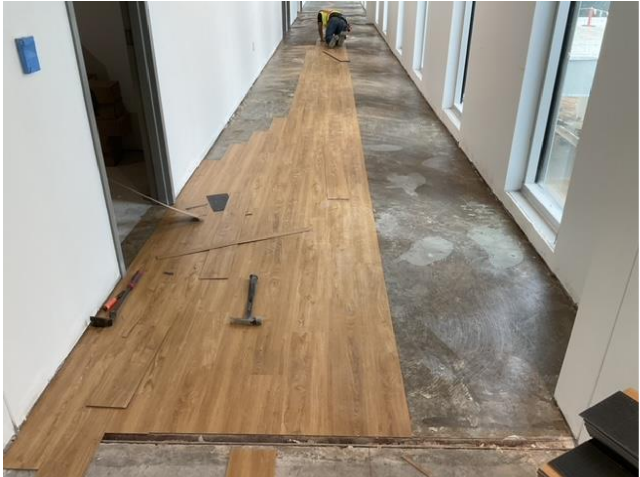
Flooring at Hallways
