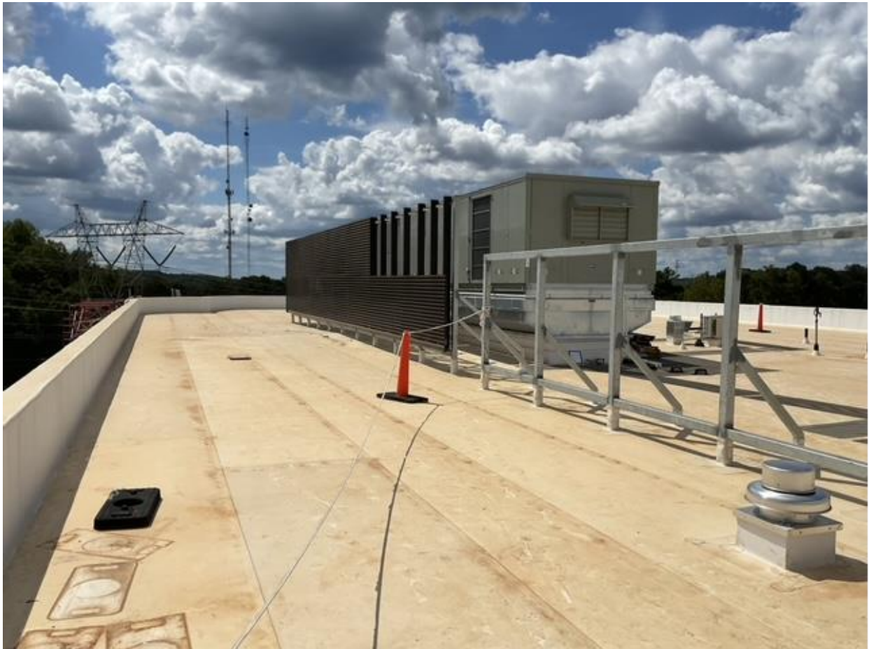
Roof Screen Install
