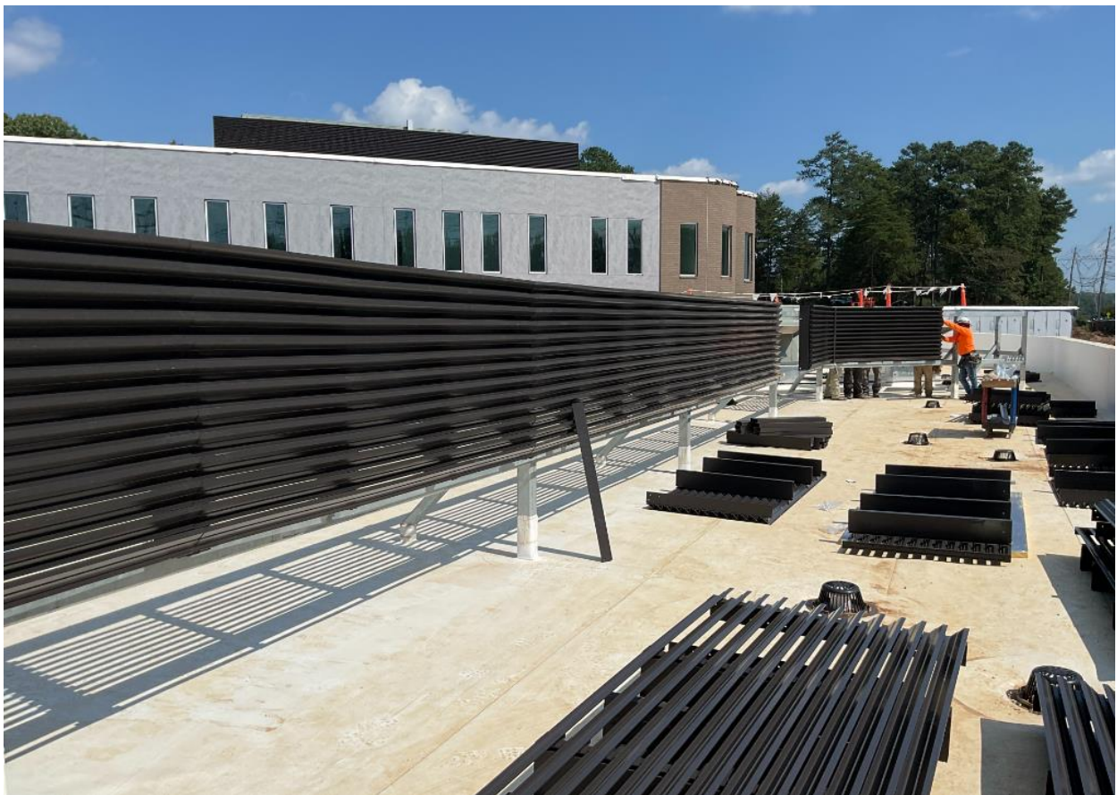
Roof Screen Install at Low Roof
