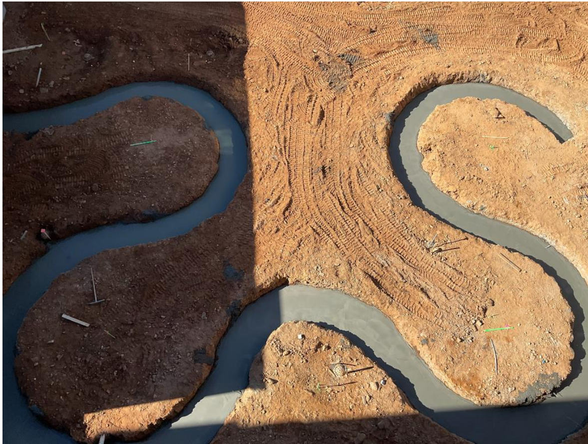
Seat Wall Footings
