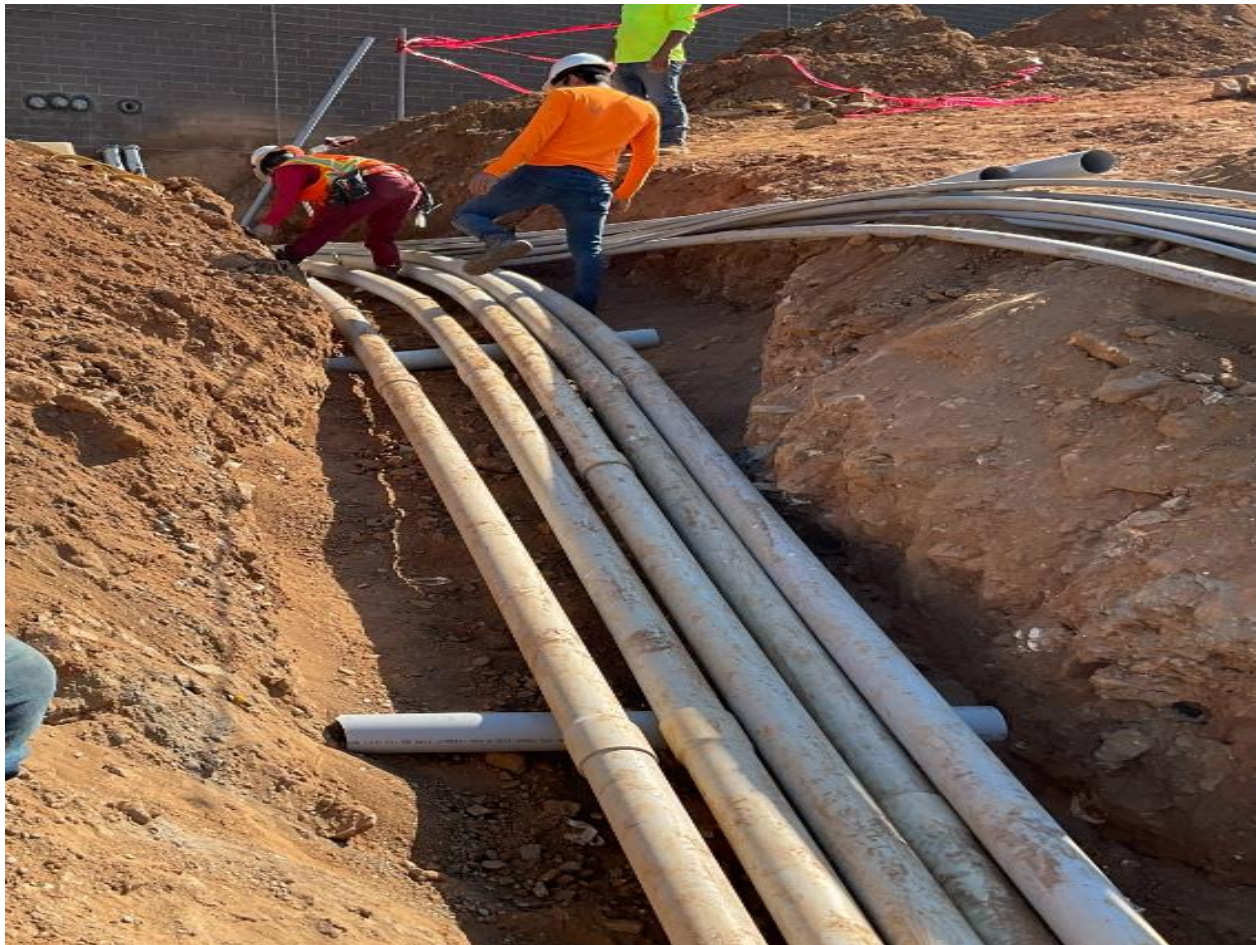
U/G Rough-In to Generator Pad
