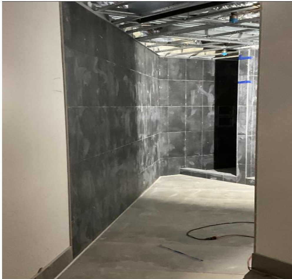
Tile at Locker Room
