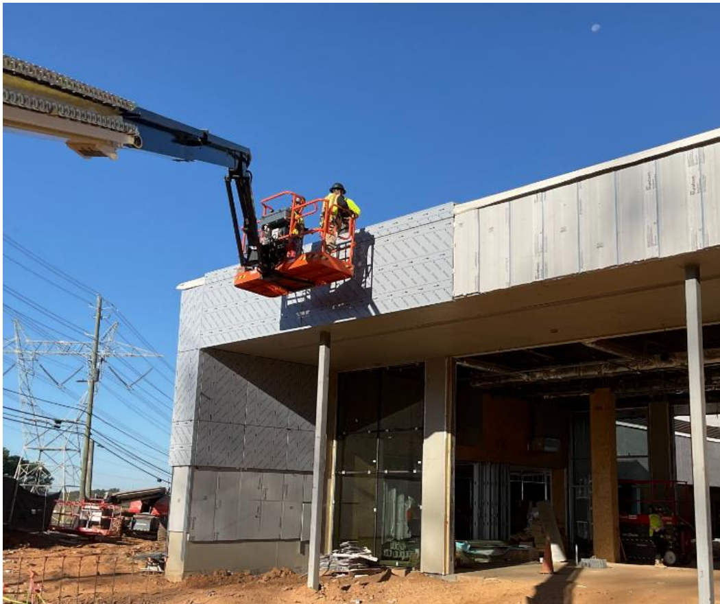
Metal Panels at Screening Area
