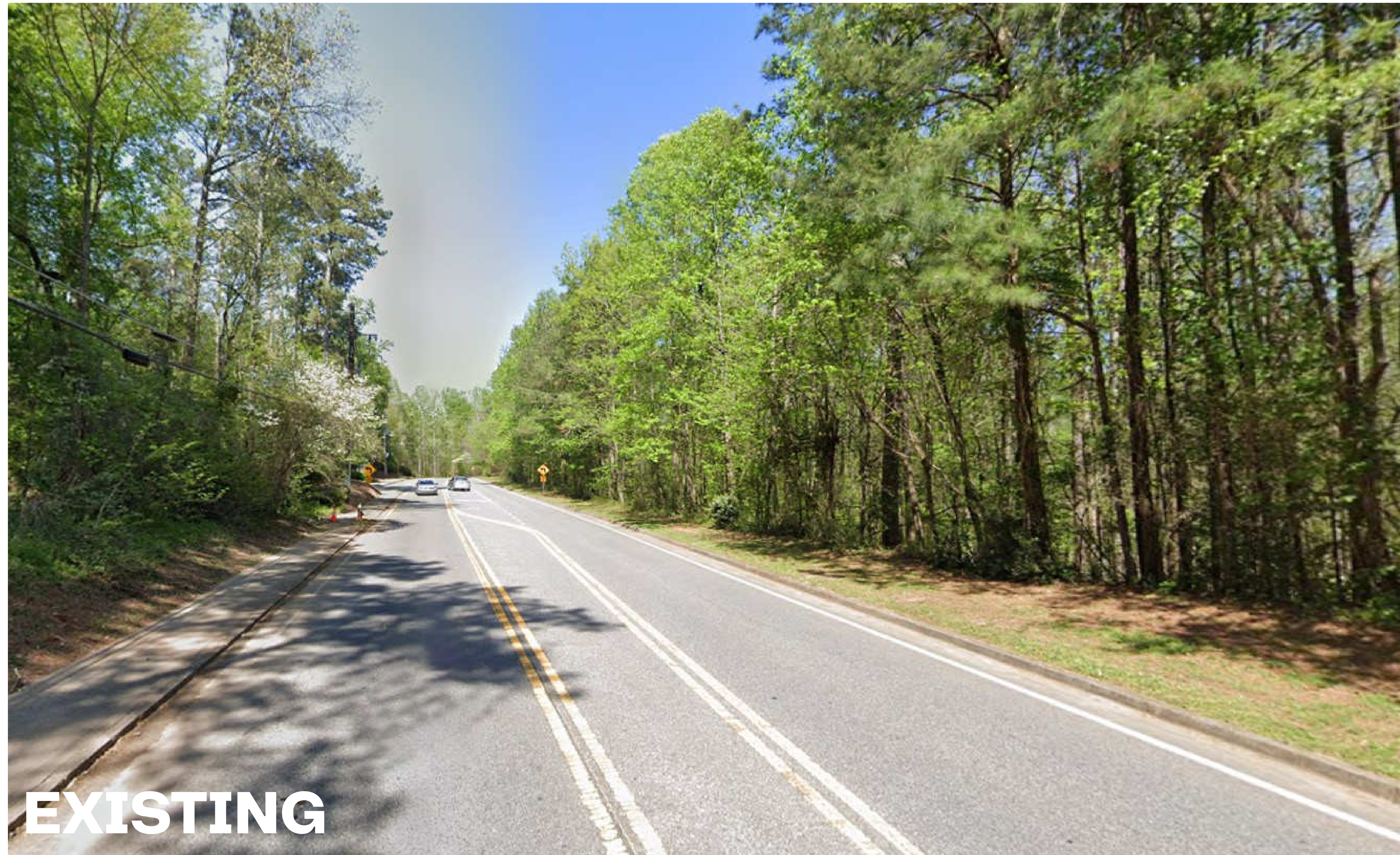
VIEW AT STA 51+50, LOOKING NORTHEAST TOWARDS SUMMER CROSSING
