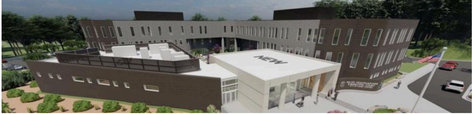
POLICE HEADQUARTERS AND COURT
