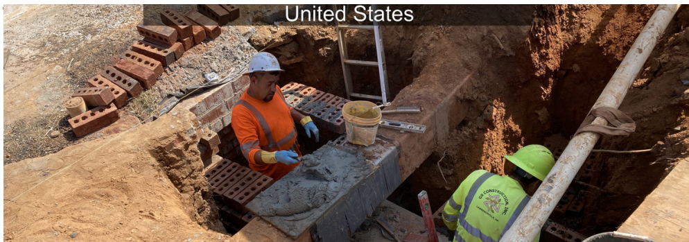
TS191 Stormwater construction and paving
