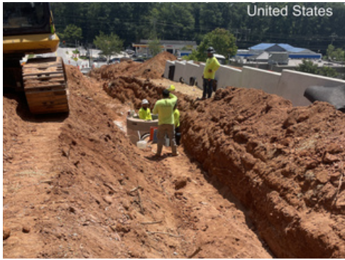
TS108 Stormwater construction
