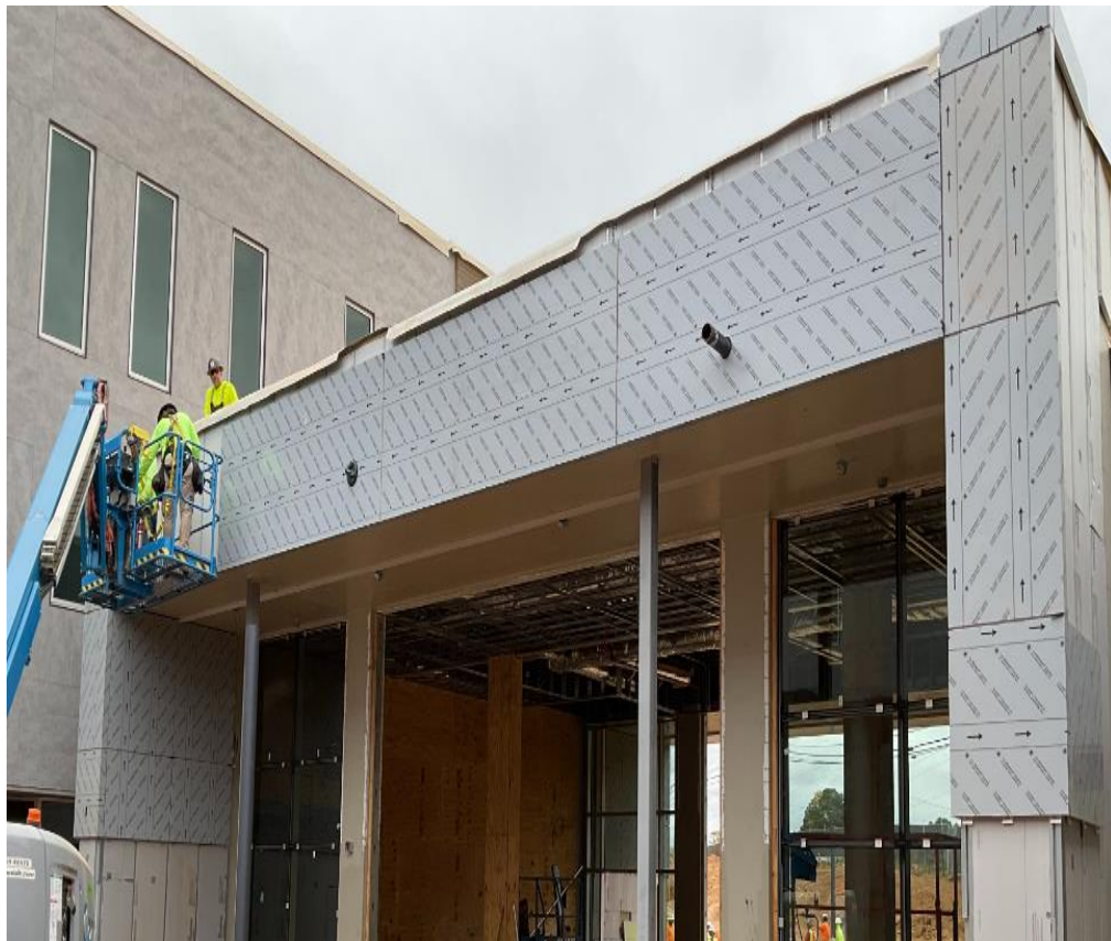
Metal Panel at Courtyard
