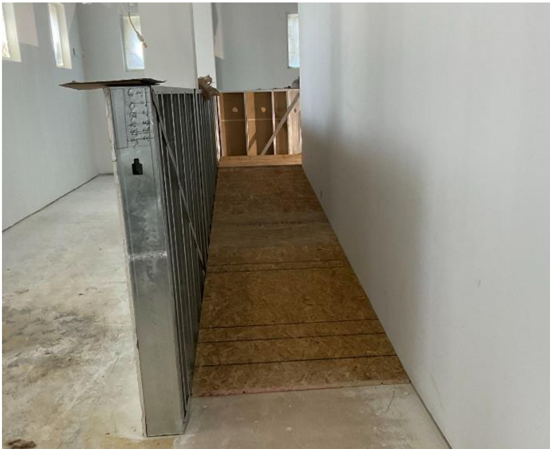
Ramp behind Judges Platform
