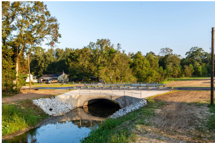
CULVERT OVER WATER BODY
