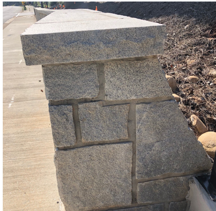
GDOT Standard Poured-in-Place Wall, Stone
