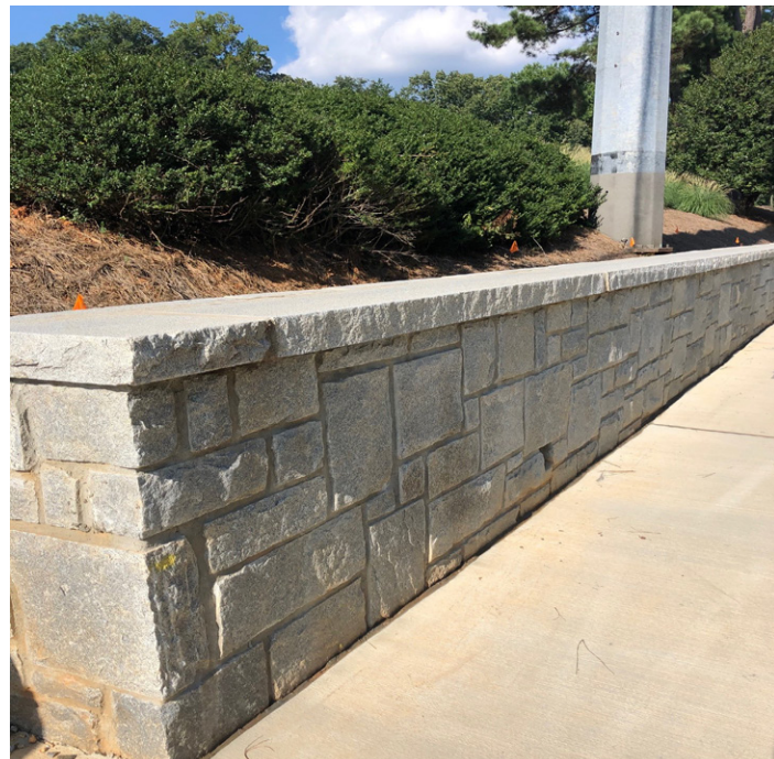
GDOT Standard Gravity Wall, Stone
