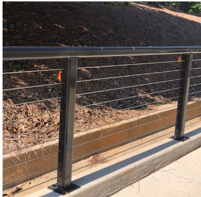
GDOT Standard 42" Cabled Handrail, Steel
