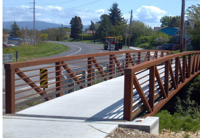
Pedestrian Bridge TrueNorth Steel
