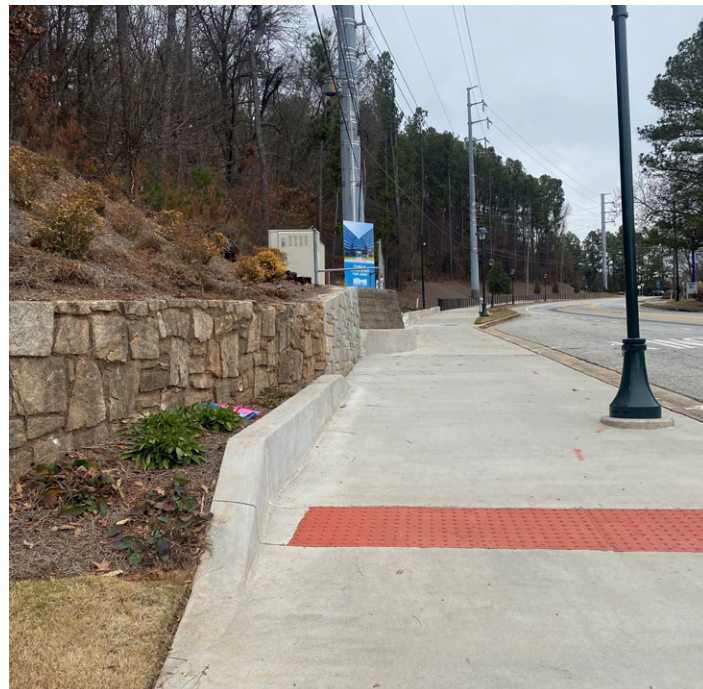
GDOT Standard Turned-Up Curb, Concrete
